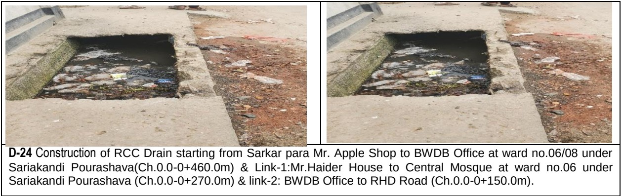
Figure 4:Existing Roads and Drains Picture
