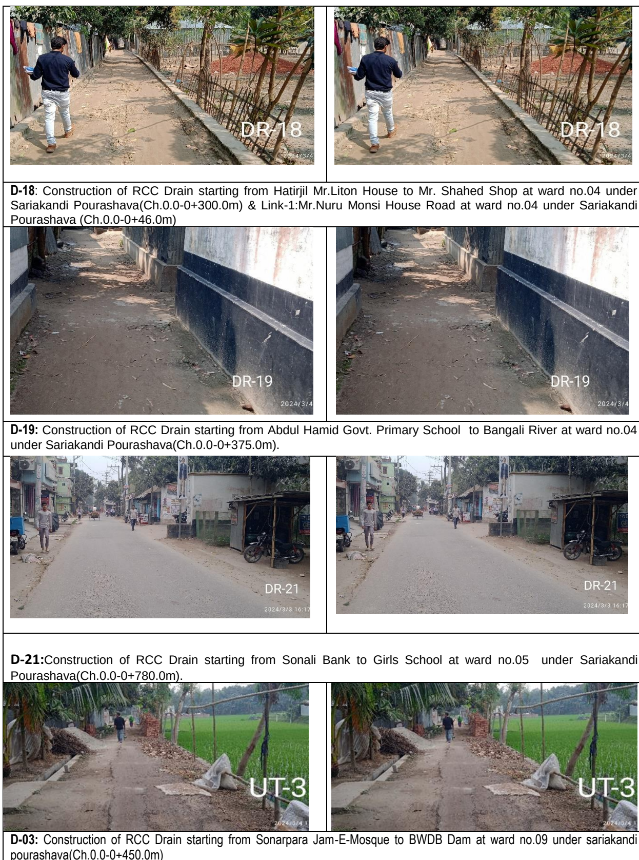
Figure 4:Existing Roads and Drains Picture
