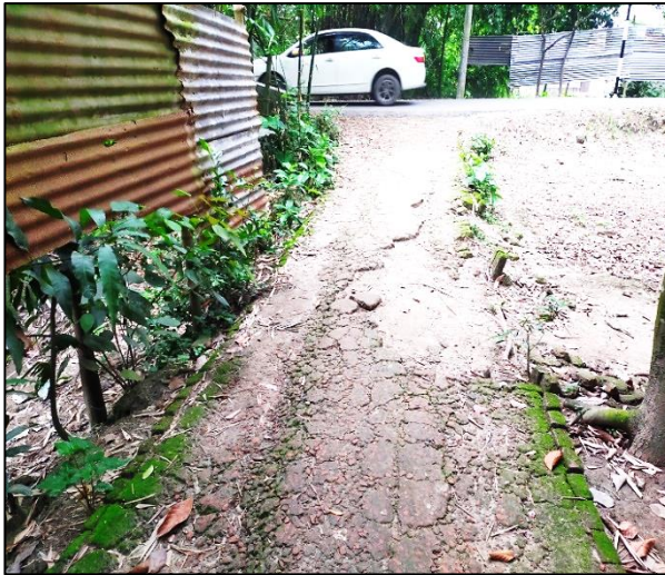
Figure 8: Some Photographs under this package
