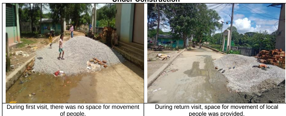
Figure 11: Temporary Placement and Removal of Construction Materials on Road Under Construction
