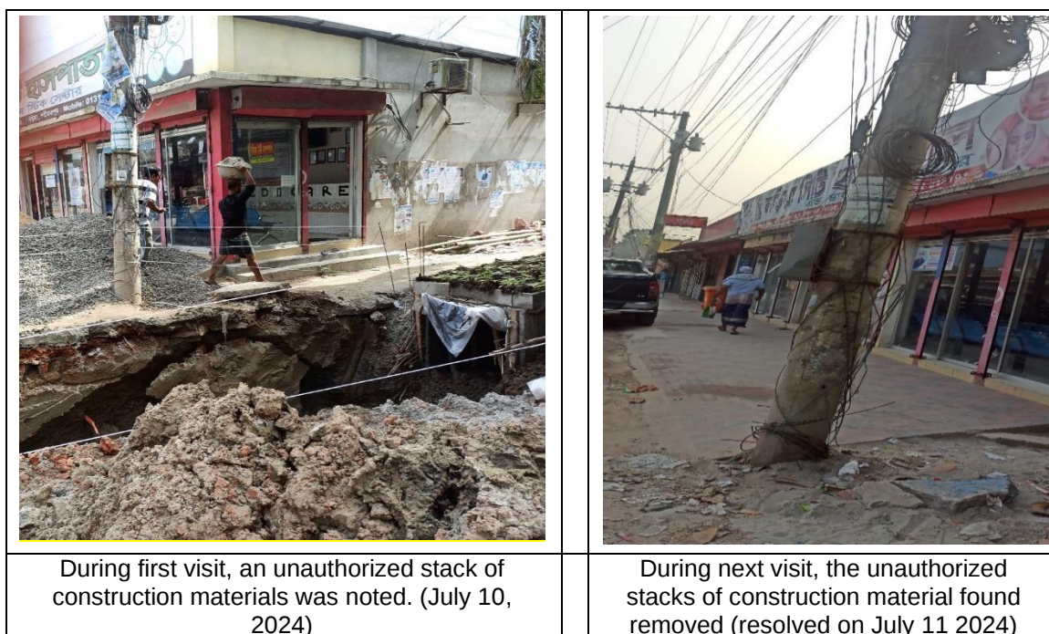
Figure 10: Construction Photos (Description below)
