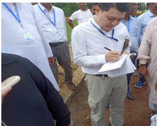
Monitoring of ongoing works at Kaliakoir
