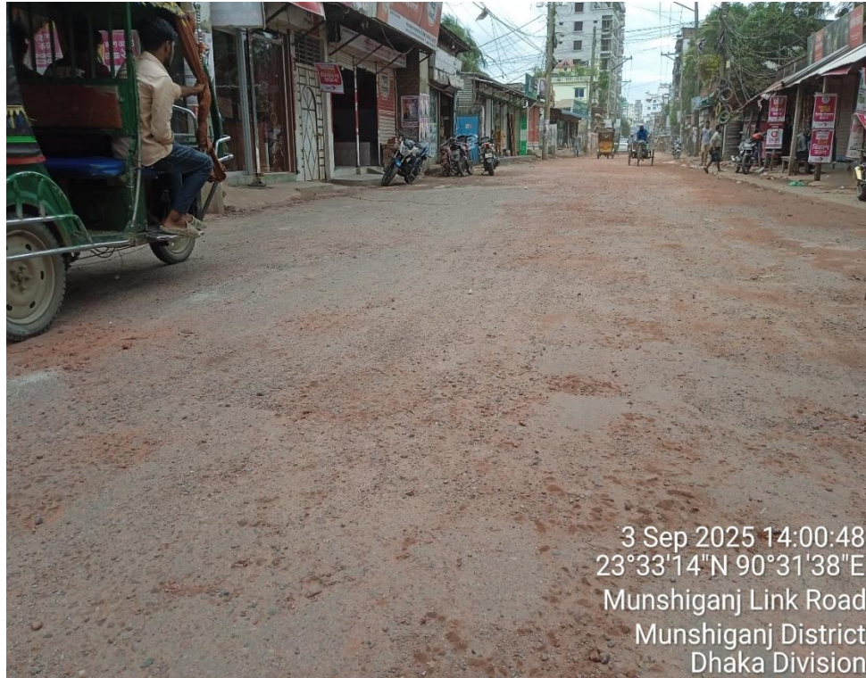
R-107 & D-75: Manikpur Ten Storied Building to Super Market Road
