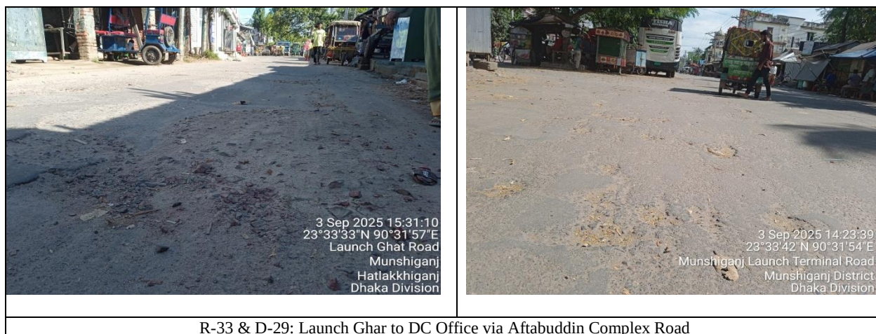
Figure 8: Some Photographs under this Package
