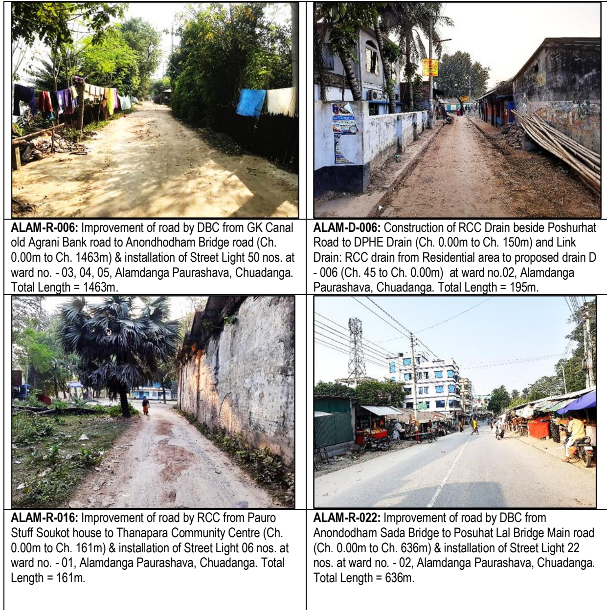
Figure 4: Existing Conditions of Pourashava Roads and Drains
