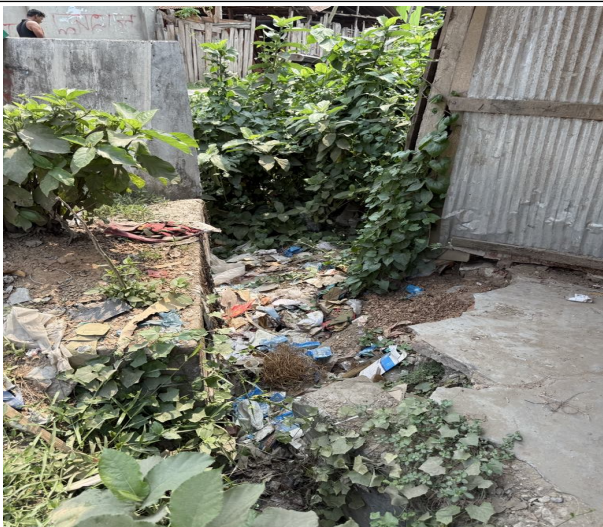
D-019:Construction of RCC Drain Starting from Anandadham Bridge to Fazlul Haque Khan Khal (Ch. 0+000 to 0+170), Toatal Length= 170min Ward no. 04 under Alamdanga Pourashava, Chuadanga.
