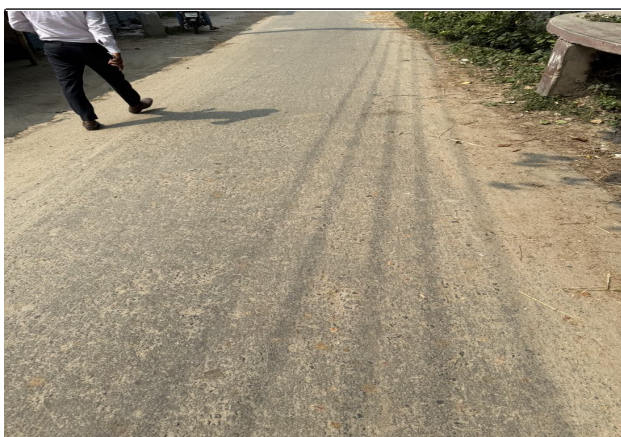
R-01.Improvement of DBC Road Starts From Earshadpur Natun Bazar to Earshadpur Academy School( Ch. 0+00 to 0+652), Total Length= 652m including Protection work 91m at ( Ch. 0+188 to 0+246, R/S), (Ch. 0+448 to 0+481, R/S), & Instalation of 23 nos. Street light in ward no. 05 under Alamdanga Pourashava, Chuadanga.
