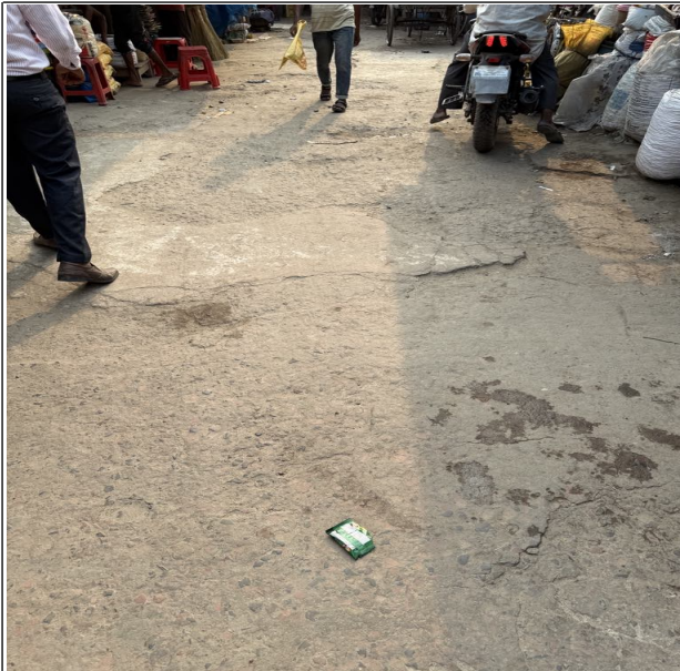
D-015:Construction of RCC Drain Starting from Canalpar Kali Mondir to Fazlul Haque Khal (Ch. 0+000 to 0+105), Total Length= 105m in ward no. 01 under Alamdanga Pourashava, Chuadanga.
