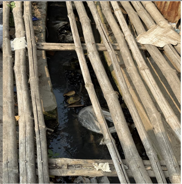
D-018:Construction of RCC Drain Starting from Horitola Mondir House to BMDF Drain via Natun Bus stand and JN Govt. school (Ch. 0+000 to 0+375), Total Length= 375m in ward no. 06 & 08 under Alamdanga Pourashava, Chuadanga.
