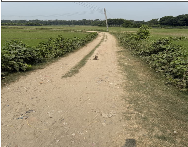
R-004 Improvement of DBC Road Starting From Infront of Ershadpur Eidgaht upto Ershadpur Aloms Garden. (Ch. 0+000 to 0+428), Total Length= 428m. & Installation of 06 nos. Street Light in Ward no. 05 under Alamdanga Pourashava, Chuadanga.
