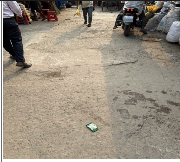
D-032:Construction of RCC Drain Starting from Komal Pal Shop of Kachari Bazar to Existi IUIDP Drain (Ch. 0+000 to 0+110), Total Length= 110m in Ward no. 02 under Alamdanga Pourashava, Chuadanga.
