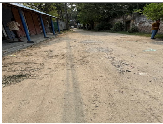
R-002: Improvement of DBC Road Starting From EarshadpurCatal Mour Edris shop to Sobed Ali Chairman House ( Ch. 0+00 to 0+872), Total Length= 872m including Protection work 57m at ( Ch. 0+416 to 0+431, R/S), (Ch. 0+666 to 0+684, L/S), (Ch. 0+735 to 0+759, R/S), 01 nos. Cross Drain (1.0m x 1.0m x 7.0m) at Ch. 605m & Instalation of 31 nos. Street light in ward no. 05 under Alamdanga Pourashava, Chuadanga.
