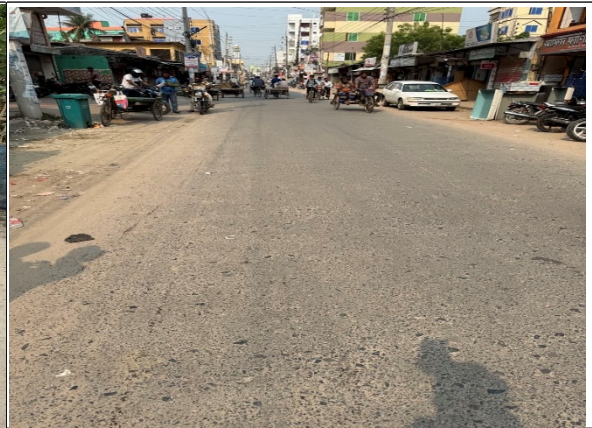
R-017: Improvement of DBC Road Starting From Chartola Sottonarayan Mondir to Ekattar Chattar via 71 Mour Towards Alamdanga Rail Station ( Ch. 0+00 to 1+411), Total Length= 1411m & Instalation of 50 nos. Street light in ward no. 01, 02 & 03 under Alamdanga Pourashava, Chuadanga.
