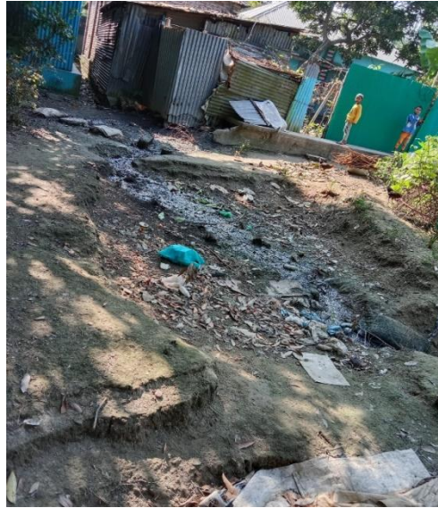
Figure IV.4: Existing Situation of Drain at Daspara LIN
