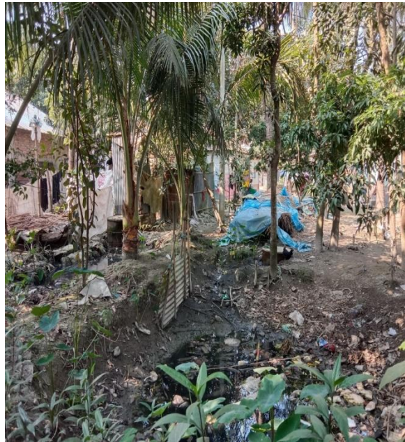
Figure IV.2: Existing Situation of Drain at Mouzzakanda LIN
