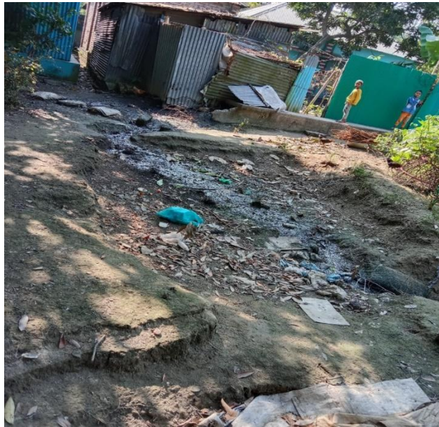
Figure IV.6: Existing Situation of Drain at Krishnapura LIN
