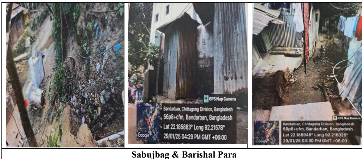
Figure IV.3: Existing Situation at Sabujbag & Barishal Para LIN
