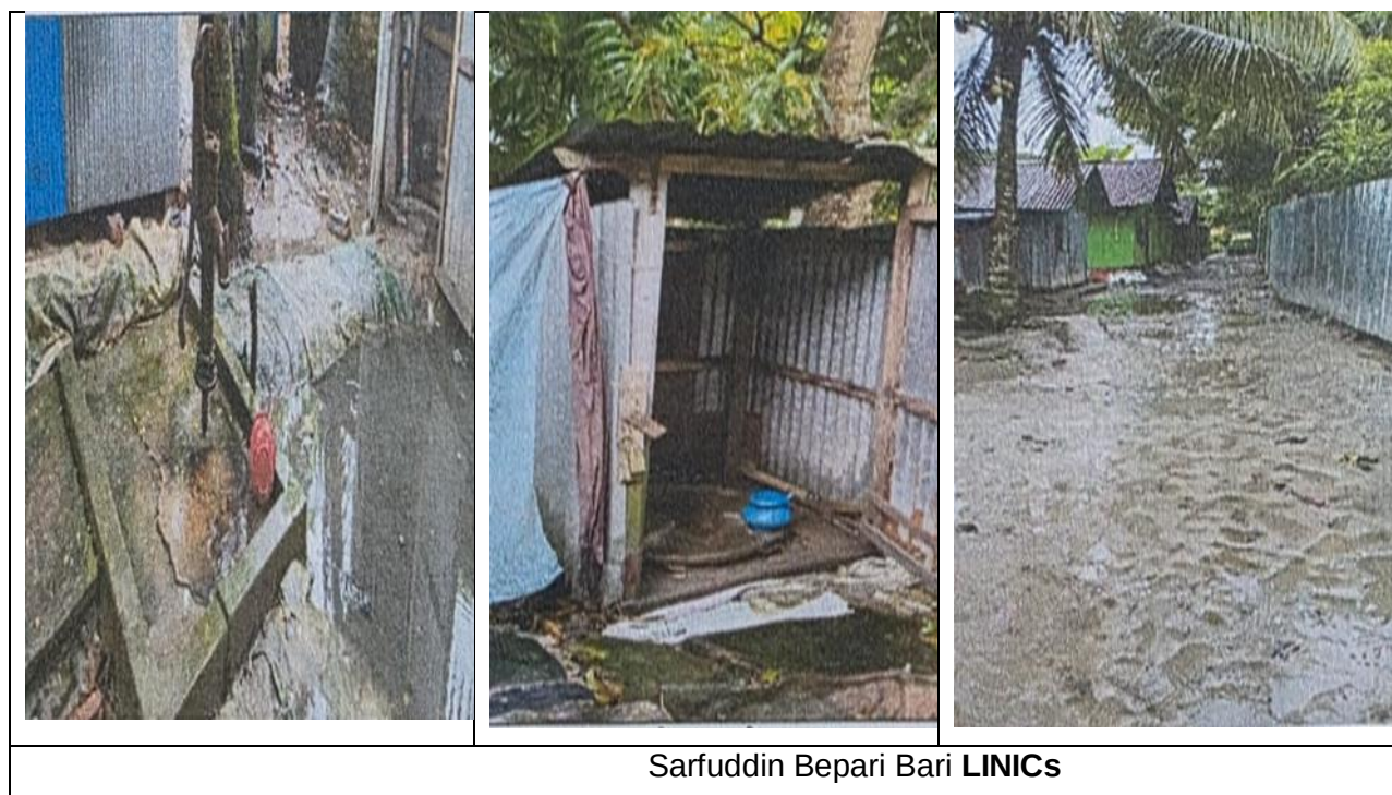
Figure IV.1: Existing Situation at Sarfuddin Bepari Bari LIN
