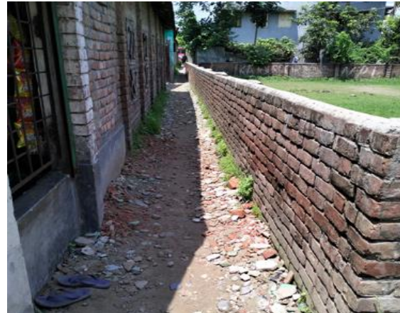
BP -D-007: Construction of RCC Drain from H/O Rezaul near Dhaka Coach Stand to Proposed drain D-11 at Farakpur Ward No.01 under Bheramara Pourashava, Kushtia.
