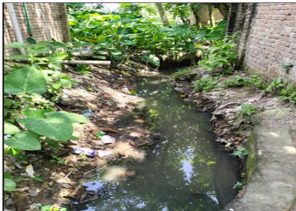
BP-D-011: Construction of RCC Drain from infront of Pourashava to existing Hazipara Lake Drain at Nawdapara & Bamonpara Ward No.03 & 09 under Bheramara Pourashava, Kushtia.
