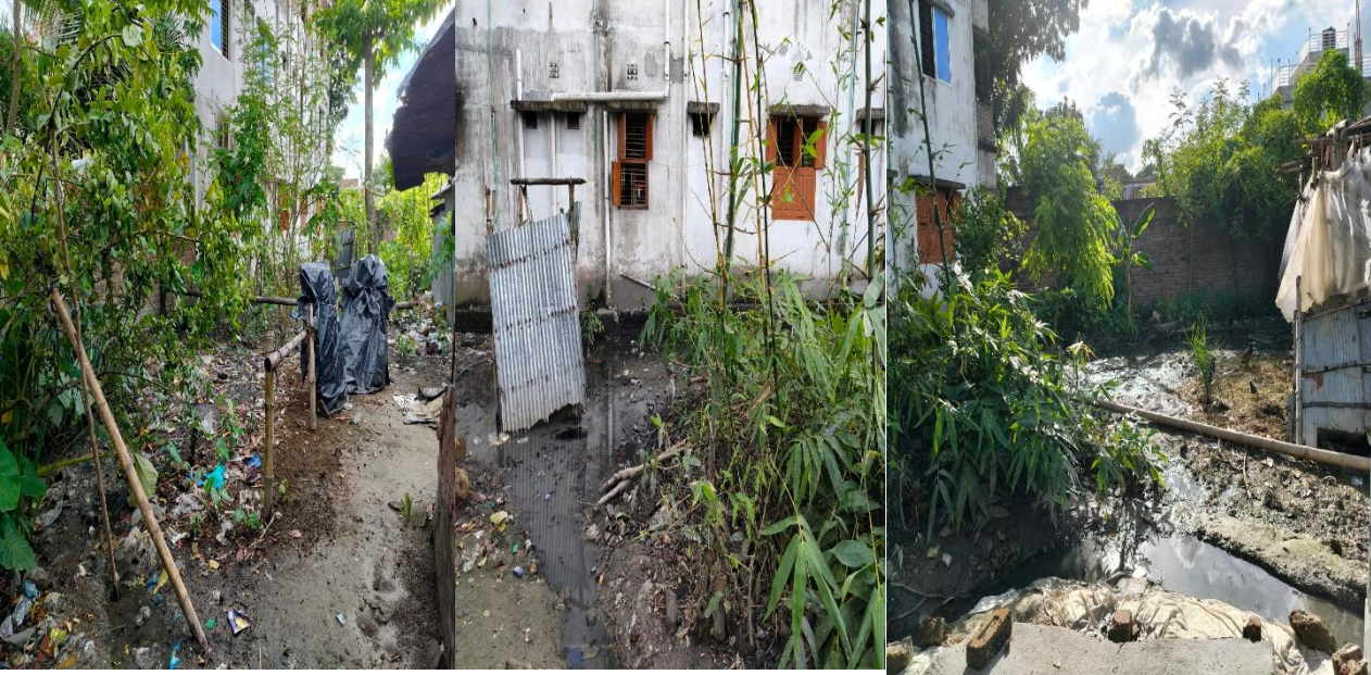
Figure IV.5: Existing Situation at Canal para LIN
