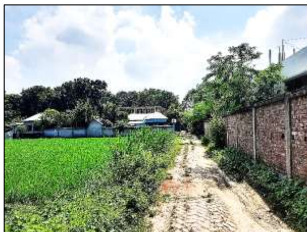
BOAL-R-005: Improvement of road by BC from East Kamargram Nurul Islam Manager house road to Raipur Mafijul house road (Ch. 0.00m to 575m) including RCC Cross Drain at Ch. 100m, Ch. 500m & installation of Street Light 20 nos. at Ward no. - 03, Boalmari Paurashava, Faridpur. Total Length = 575m.
