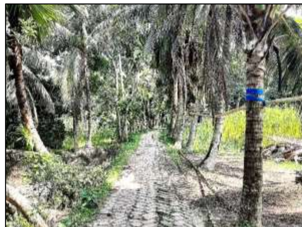
BOAL-R-004: Improvement of road by BC from East Kamargram Kamal Shop to the H/O Alep Kha via Lutfur Mridha house road (Ch. 0.00m to 855m) including RCC Cross Drain at Ch. 300m, Protection Workat Ward no. - 03, Boalmari Paurashava, Faridpur. Total Length = 855m.
