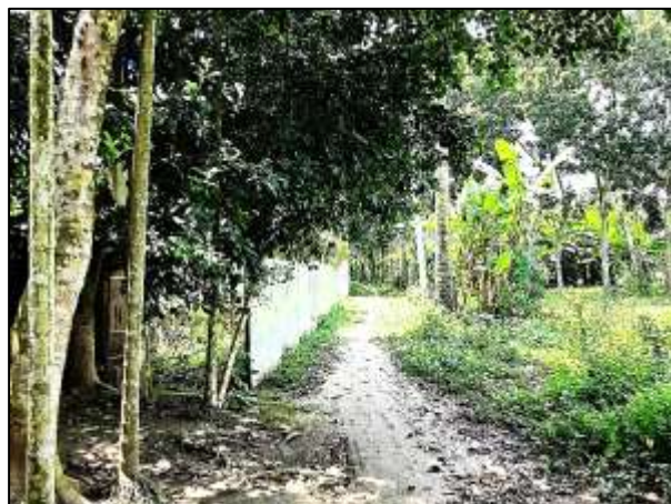
BOAL-R-003: Improvement of road by RCC from Gunboha Alamin house near Beribadh to Khayer Sheikh house road via Kundubari road (Ch. 0.00m to 400m) & installation of Street Light 14 nos. at Ward no. -01, Boalmari Paurashava, Faridpur. Total Length = 400m.
