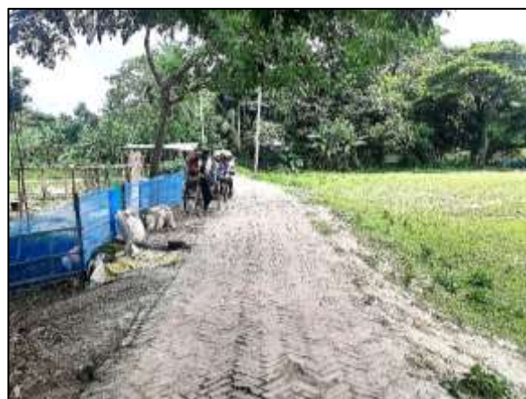
BOAL-R-010: Improvement of road by BC from R&H road near H/O Sanjit to H/O Siddiq Councilor near road via Nannu Councilor (Ch. 500.00m to 752m) & installation of Street Light 9 nos. at Ward no. - 06 & 07, Boalmari Paurashava. Total Length = 252m.
