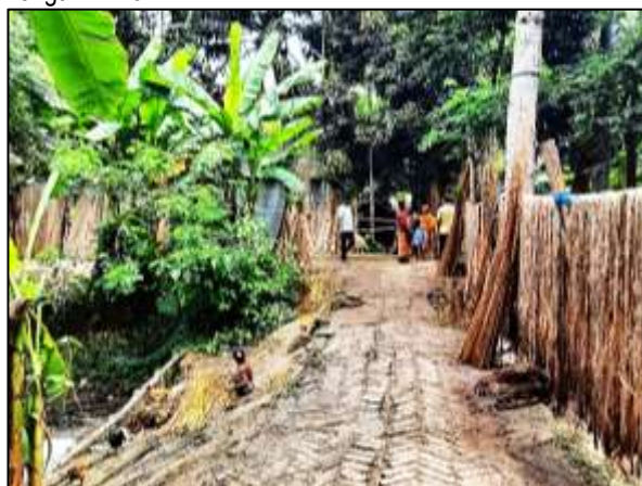
BOAL-R-011: Improvement of road by BC from Moddergati, Moddergati Malek Sikder house to Saheb Ali house via Moddergati Graveyard road (Ch. 0.00m to 410m) & installation of Street Light 15 nos. at Ward no. - 07, Boalmari Paurashava. Total Length = 410m.
