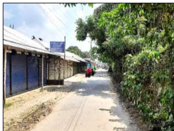
BOAL-R-002: Improvement of road by Dense Bituminous Carpeting starting from Shibpur Sanowar Shop to Boalmari Rail Way Station (Ch. 0.00m to 485m) including Protection Work at (Ch. 15m to 45m, R/S), (Ch. 332m to 450m, L/S) at Ward no. - 05, Boalmari Paurashava, Faridpur. Total Length = 485m.
