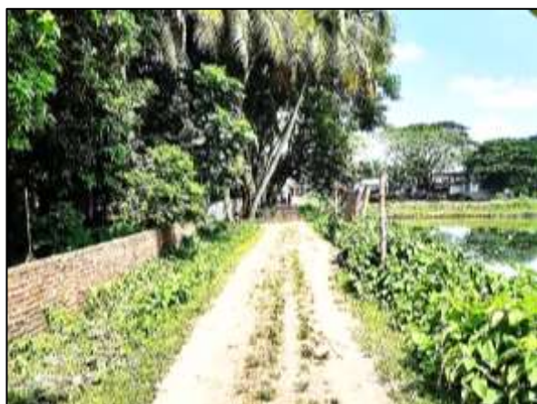
BOAL-R-009: Improvement of road by RCC from West Solna Farid Mia house to Nagor Mia Hauque house (Ch. 0.00m to 215m) including Protection Work at (Ch. 5m to 39m, L/S), (Ch. 45m to 215m, B/S) & installation of Street Light 8 nos. at Ward no. - 06, Boalmari Paurashava. Total Length = 215m.
