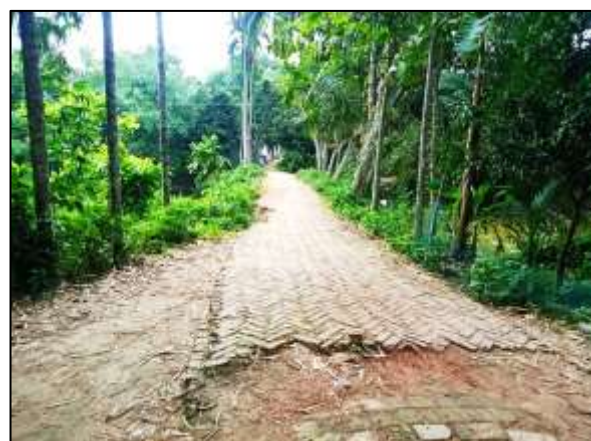
BOAL-R-008: Improvement of Sotashi road by DBC, Thakurpur road to Rail Line via Sotashi Momin market, Kala Sheikh house (Ch. 0.00m to 765m) including Protection Work at (Ch. 239m to 290m, L/S), (Ch. 670m to 700m, L/S), (Ch. 735m to 765m, R/S) & installation of Street Light 27 nos. at Ward no. - 04, Boalmari Paurashava. Total Length = 410m.
