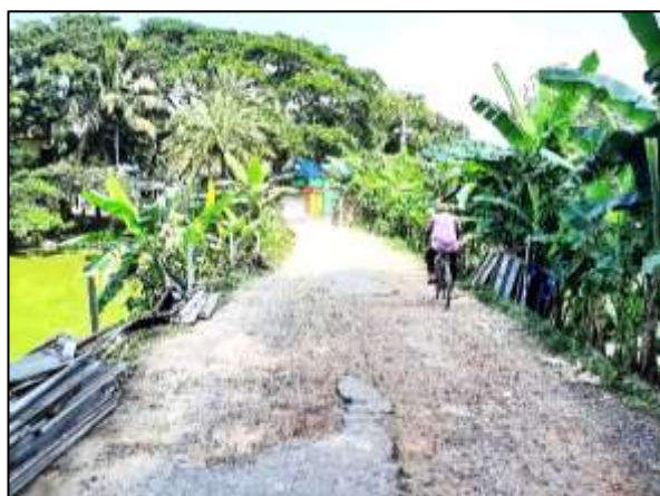
BOAL-R-001: Improvement of Road by Dense Bituminous Carpeting (DBC), starting from Kamargram Panjery Academy to end of East side Paurashava border via Govt. College (Ch. 0.00m to 1350m) including Protection Work at (Ch. 620m to 710m, L/S) at Ward no. - 05, Boalmari Paurashava, Faridpur. Total Length = 1350m.
