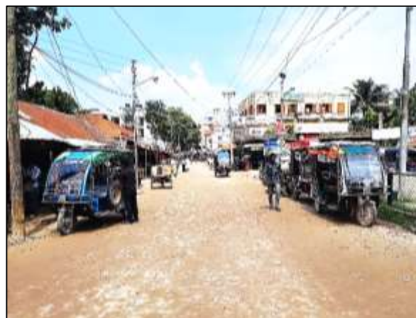
BOAL-D-004: Construction of RCC Drain from Boalmari Chowrasta to Govt. College Gate proposed drain D - 003 via Rail Station (Ch. 935m to 0.00m) at Ward no. - 05, Boalmari Paurashava, Faridpur. Total Length = 935m.
