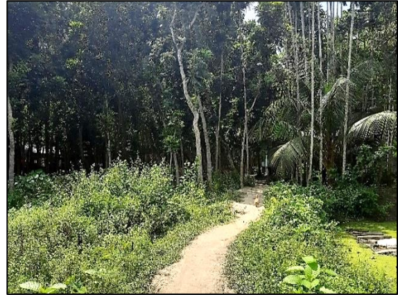
BOAL-R-023: Improvement of Road by RCC from Abu Kalam Mill to Gorai Chand Mazar Monch (Ch. 0.00m to Ch. 220m) Protection Work at (Ch. 5m to 41m, B/S) & installation of Street Light 08 nos. at Ward no.- 09, Boalmari Pourashava, Faridpur. Total Length = 220m.
