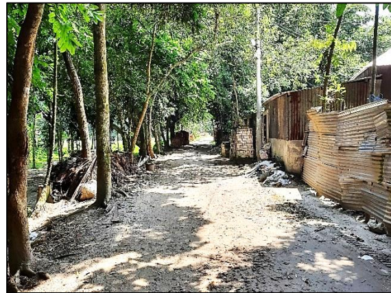
BOAL-R-036: Improvement of Road by DBC from Gunbaha near Shajahan house road to Akram Member House road (Ch. 0.00m to Ch. 1250m) & installation of Street Light 43 nos. at Ward no. - 01, Boalmari Pourashava, Faridpur. Total Length = 1250m.
