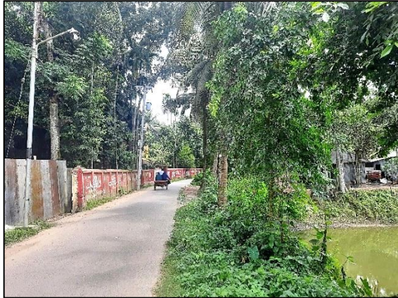
BOAL-R-021: Improvement of Road by DBC from Boalmari Food Go down to Solna Govt. Primary School (Ch. 0.00m to Ch. 880m) at Ward no. - 06 & 07, Boalmari Pourashava, Faridpur. Total Length = 880m.
