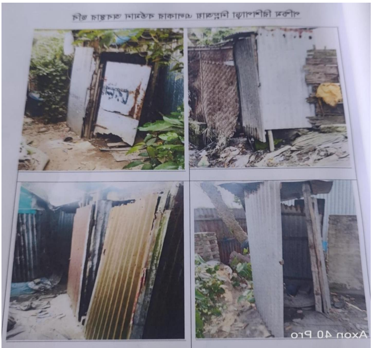
Figure IV.4: Existing Situation at Paschim Rishi Para LIN
