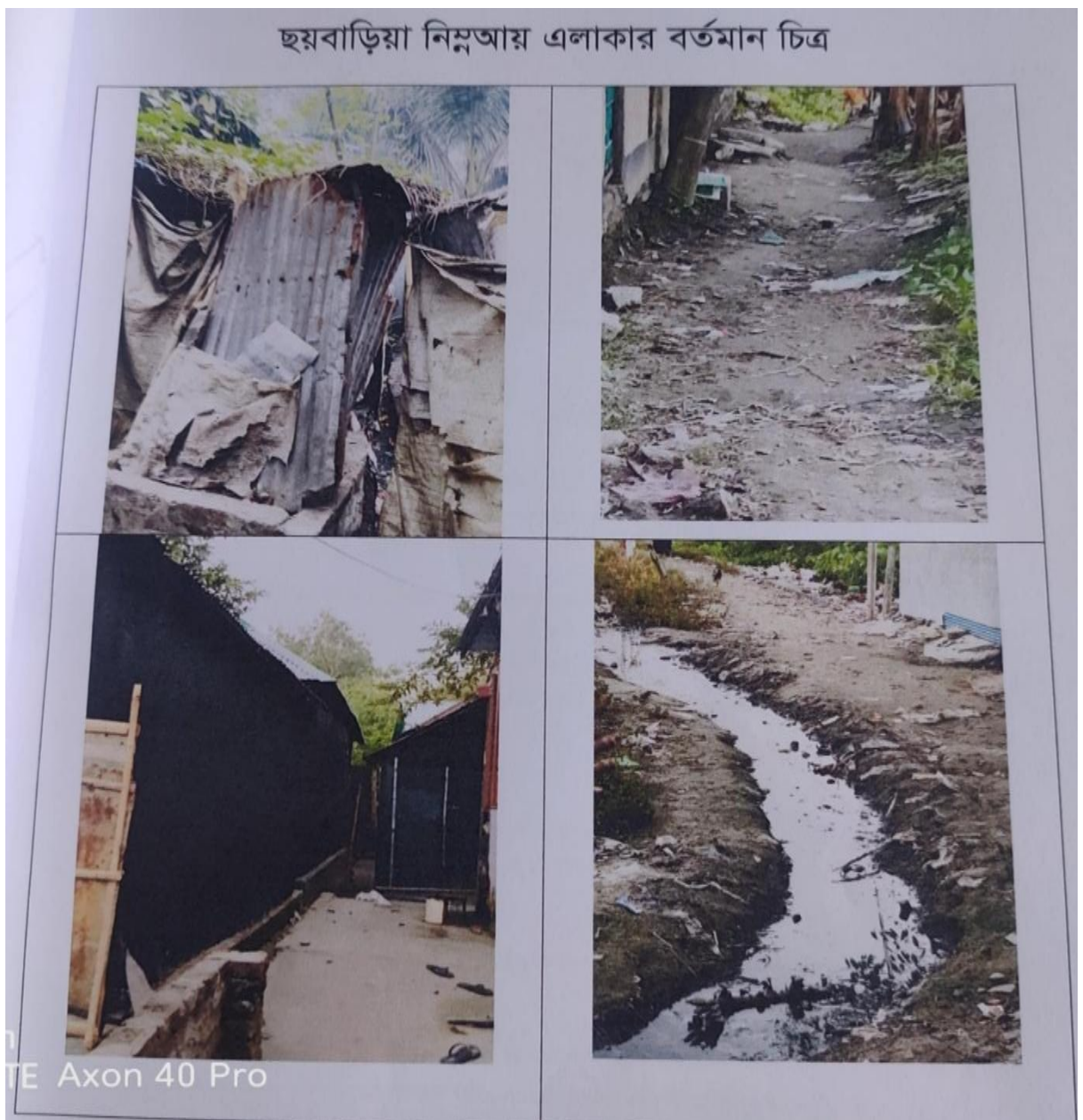
Figure IV.5: Existing Situation at Choybaria Gram LIN
