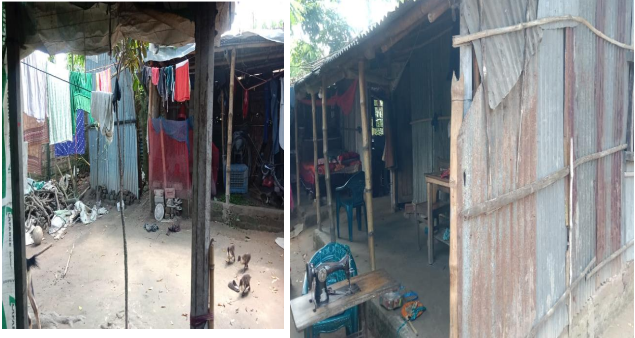
Figure IV.3: Existing Situation at Paschim Rishi Para LIN
