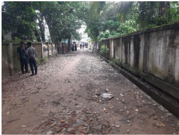
CHUN-R-006: "Improvement of Road by Reinforced Cement Concrete (RCC), starting from Balla road to Forest Office via Post Office (Ch. 0.00m - 90.00m), including RCC Cross Drain at Ch. 50m, at Ward no.- 6, Chunarughat Paurashava, Habiganj. Total Length = 90m."
