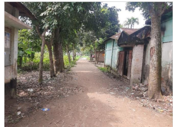
CHUN-R-022: "Improvement of Road by Reinforced Cement Concrete (RCC) at Hatunda, starting from Shotong road to Telutta road (Ch. 0.00m - Ch. 571.00m), including RCC Cross Drains at Ch. 0m & Ch. 551m, Protection Works at (Ch. 500m to Ch. 535m, R/S) and installation of Street Lights of 20 nos., at Ward no.- 3, Chunarughat Paurashava, Habiganj. Total Length = 571m."
