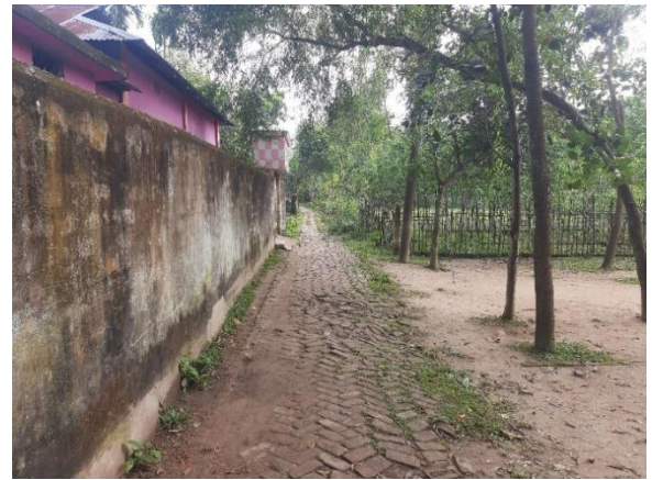
CHUN-R-007: "Improvement of Road by Reinforced Cement Concrete (RCC) at Pakuria, starting from Talukder Bari road to Zumma Mosque road via Kashem Miah's house (Ch. 0.00m - Ch. 428.00m), including RCC Cross Drain at Ch. 291m, Protection Works at (Ch. 212m to Ch. 235m, L/S) and installation of Street Lights of 15 nos., at Ward no.- 7, Chunarughat Paurashava, Habiganj. Total Length = 428m."
