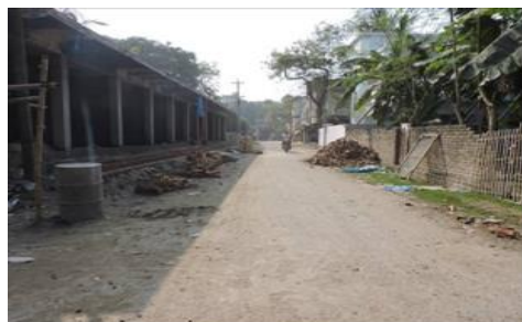
D-02: Construction of RCC Drain beside Mohi Master House to Mosarof Derection House road D-02 (ch. 0+000-0+254km)
