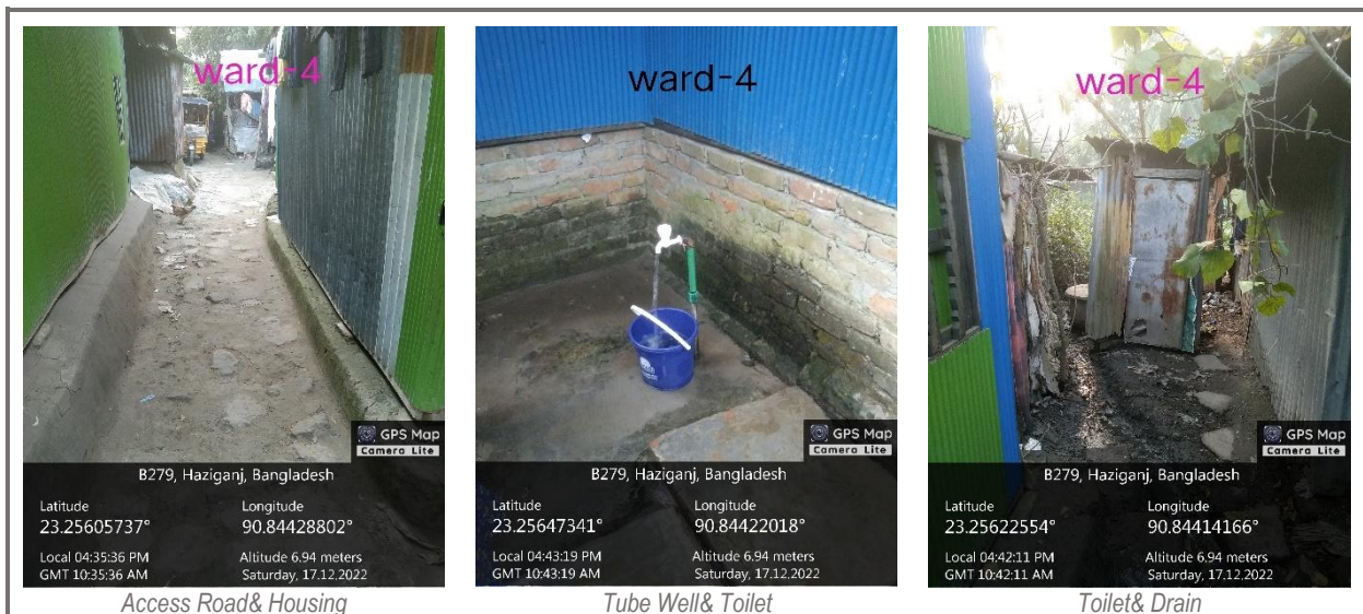
Figure IV.2: Existing Situation at Mokimabad Gain Bari LIN
