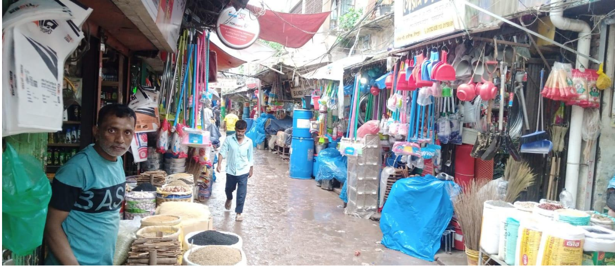
D-06: Construction of RCC Drain Starting from Haziganj Bazar Torkari Potti to Dakatia River (Ch. 0.00-210.00m) at Ward no-06, Haziganj Paurashava, Chandpur (Total Length=210.00m).
