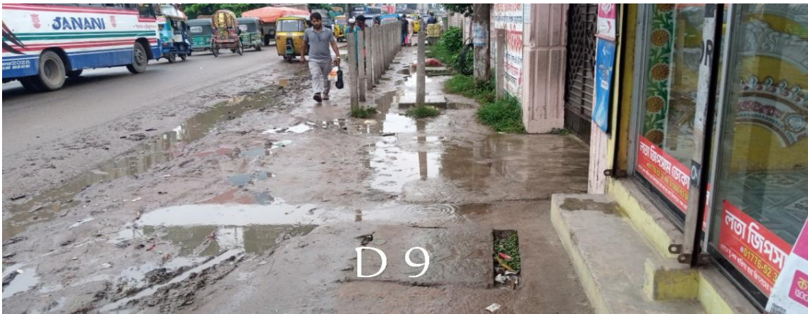
D-09: Construction of RCC Drain Starting from Beside Cumilla-Chadpur Road to Dakatia River via Mokimabad Ashram (Ch. 0.00-580.00m) at Ward no-05, Haziganj Paurashava, Chandpur (Total Length=580.00m).
