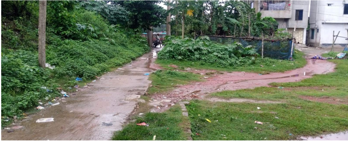
D-011:Construction of RCC Drain Starting from Mokimabad Late Md. Akub Ali Mozumder house to Existing Drain (Ch. 0.00-193.00m) & Link drain (Ch. 0.00 to 200.00m) Total Length=393.00m in Ward no-04, under Haziganj Paurashava, Chandpur.
