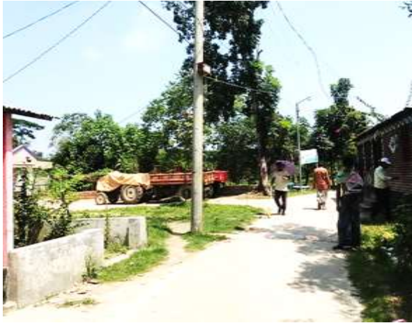
HOSS-D-007: Construction of RCC drain adjacent to the Road starting from the Upazilla Model Mosjid to the house of Late Habibur Rahman (Ch. 0.00m - Ch. 451.00m), at Ward no- 5, Hossainpur Pauashava, Kishoreganj.
