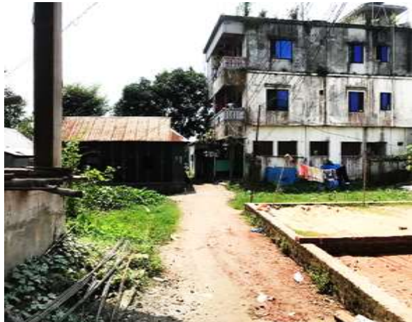
HOSS-D-024: Construction of RCC Drain starting from Himu-Shimu Pharrmacy adjacent to Shahid Syed Nazrul Islam Sarani to h/o Toufique (Ch. 0.00m – Ch. 120m), at Ward no.- 7, Hossainpur Paurashava, Kishoreganj.
