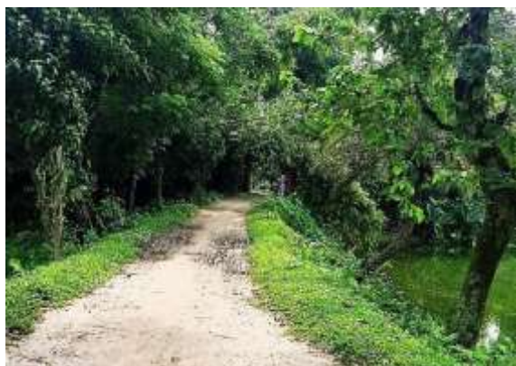
KALI-R-004: Improvement of road by DBC from Gang Shing Mour to Vataria Bridge at Chowra Nayabari road (Ch. 0.00m to 950m) including Protection Work at (Ch. 103m to 137m B/S), (Ch. 275m to 375m, L/S) & installation of Street Light 33 nos. at Ward No. - 7, Kaliakair Paurashava, Gazipur. Total Length = 950m
