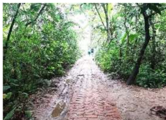
KALI-R-008: Improvement of road by DBC (a) from Kaliakair - Kapashia road near Peerbari to Durbati Govt. Primary School and (b) Link Road -1 from Al Falah Mosque to Bokterpur road including Protection Work & installation of Street Light 42 nos. at Ward No. - 1, Kaliakair Paurashava, Gazipur. Total Length = 1200m
