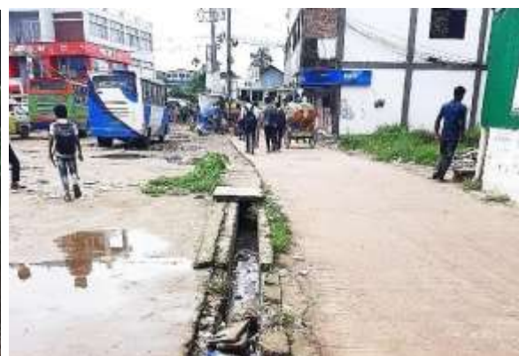
KALI-D-005: Construction of RCC Drain from Monshurpur Madinatul Monowara Madrasah to Shitolokkha River via Kaliakair Pilot School (Ch. 0.00m to 536m) at Ward no. - 04, Kaliakair Paurashava, Gazipur. Total Length = 536m
