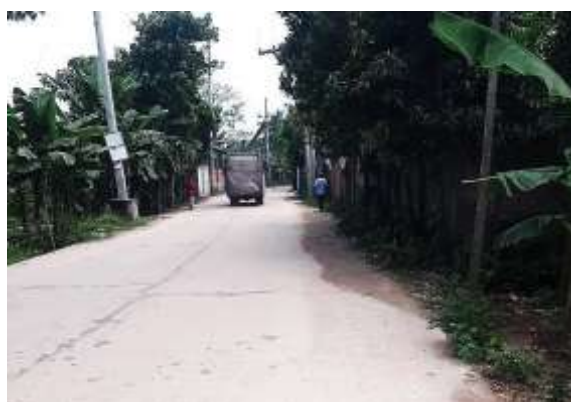
KALI-D-004: Construction of RCC Drain from RFL Gate (Gate no - 09) at Mulgaon Khal, (Ch. 0.00m to 525m) at Ward no. - 08, Kaliakair Paurashava, Gazipur. Total Length = 525m
