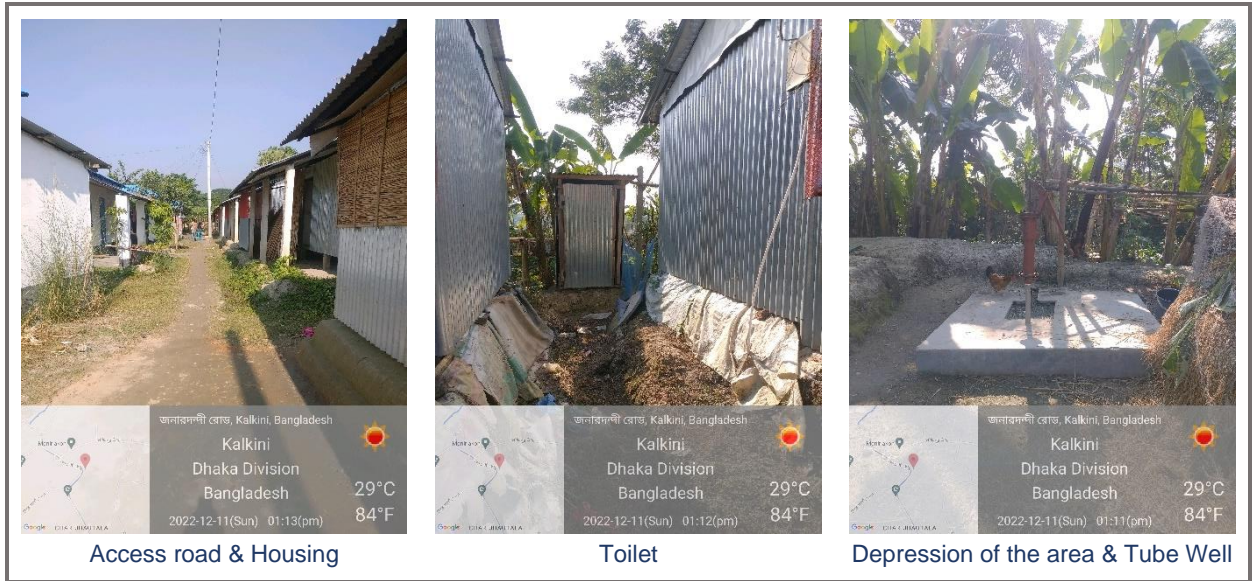
Figure IV.1: Photographs of Existing Conditions of Lamchori LIN
