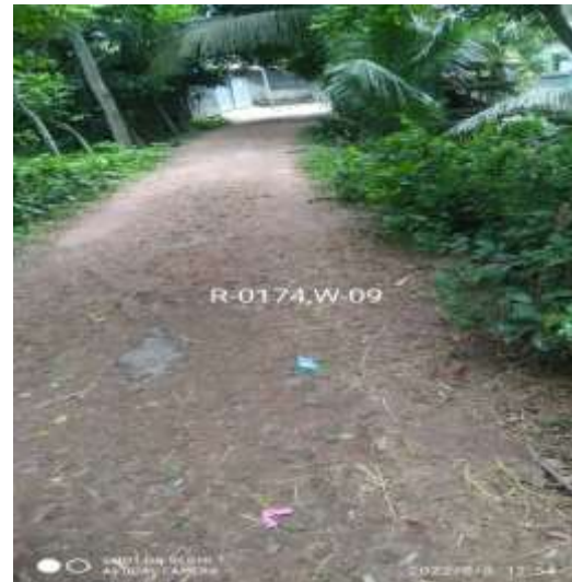
KALK-R-174: Improvement of road by RCC from Dhaka Barishal Highway Sadar Ashram to Kazi Bari Gopalpur BC road including Protection Work at (Ch. 20m to 50m, L/S), (Ch. 210m to 240m, L/S), (Ch. 220m to 250m, R/S) & installation of Street Light 20 nos. at Ward no - 9, Kalkini Pourashava, Madaripur. Total Length of road = 545m.
