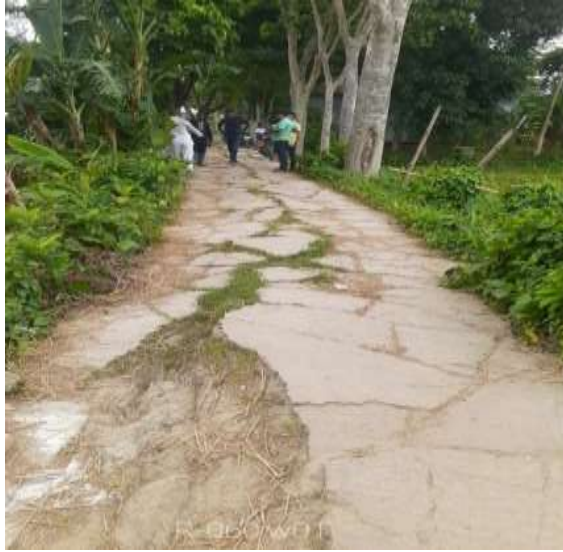
KALK-R-060: Improvement of road by RCC from Dokkhin Rajdi GPS to Khokan Hawlader house including RCC Box Culvert at Ch. 400m & installation of Street Light 23 nos. at Ward no - 1, Kalkini Pourashava, Madaripur. Total Length = 665m.
