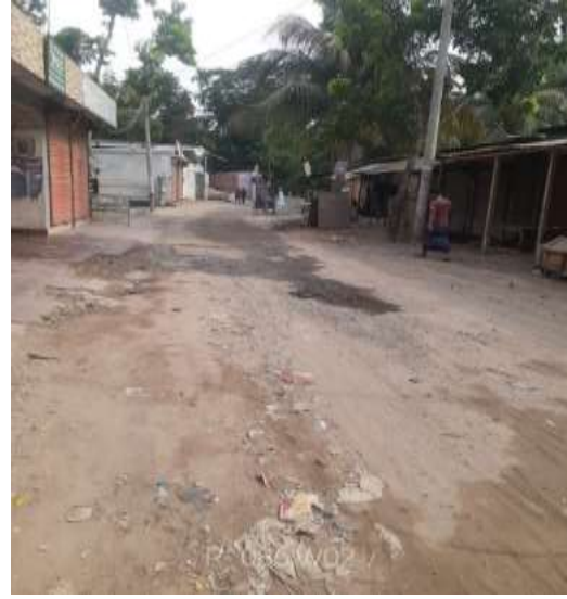
KALK-R-086: Improvement of road by Dense Bituminous Carpeting from Kalkini Mach Bazar to Dokkhin Thengamara Khokan Bepari house road including Protection work at (Ch. 255m to 275m, L/S), (Ch. 450m to 500m, B/S), (Ch. 1320m to 1365m, L/S) & installation of Street Light 61 nos. at Ward no - 2, Kalkini Pourashava, Madaripur. Total Length = 1800m.
