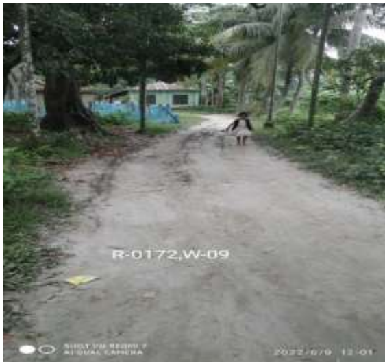
KALK-R-172: Improvement of road by Dense Bituminous Carpeting (a) from Bir Mohon Road Engr. Miraz house to Gopalpur Jame Masjid, (b) Link road - 1, Masudur Rahman road, (c) Link road - 1, (d) Link road - 2, Engr. Limon house road including Protection Work at (Ch. 120m to 140m, B/S), (Ch. 200m to 310m B/S), (Ch. 90m to 180m, L/S), (Ch. 120m to 160m, R/S), (Ch. 50m to 80m, R/S) & installation Street Light 28 nos. at Ward no - 9, Kalkini, Total Length = 735m.
