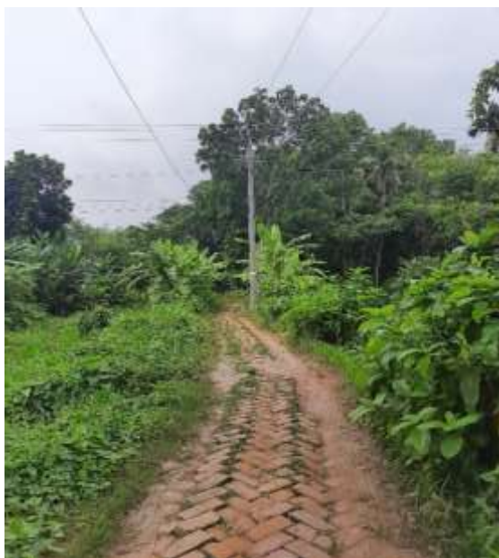
KALK-R-01: Improvement of road by RCC from Kalkini - Vurghata (Vobotosh Datta) road to Anowar Sikder house road including RCC Cross Drain at Ch. 250m, RCC Box Culvert at Ch. 350m, Protection Work at (Ch. 75m to 95m, B/S), (Ch. 350m to 400m, R/S), & installation of Street light 17 nos. at Ward no - 1, Kalkini Paurashava, Madaripur. Total Length = 480m
