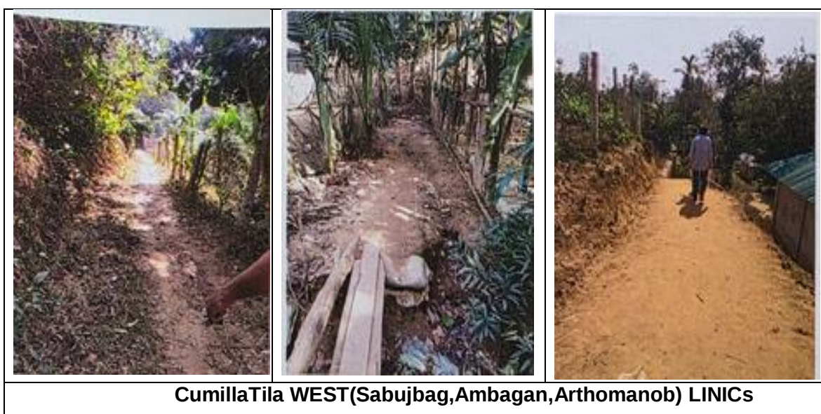
Figure IV.4: Existing Situation at Cumilla Tila WEST(Sabujbag,Ambagan,Arthomanob) LIN
