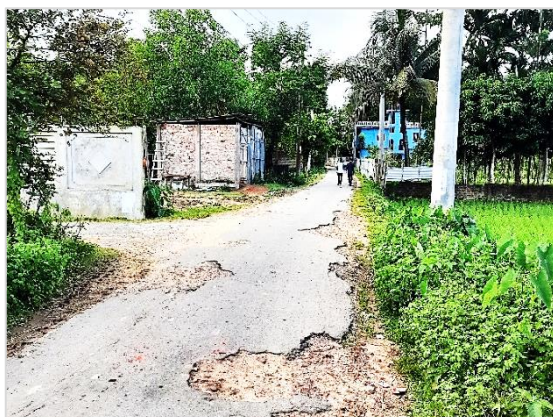
KULA-R-014: Improvement of road by RCC from RHD road Near Alalpur School at Chatalgaon towards north direction up to Kulaura - Nawabganj Road (Ch. 0.00m to Ch. 1330m) at Ward no. - 08, Kulaura Paurashava.
