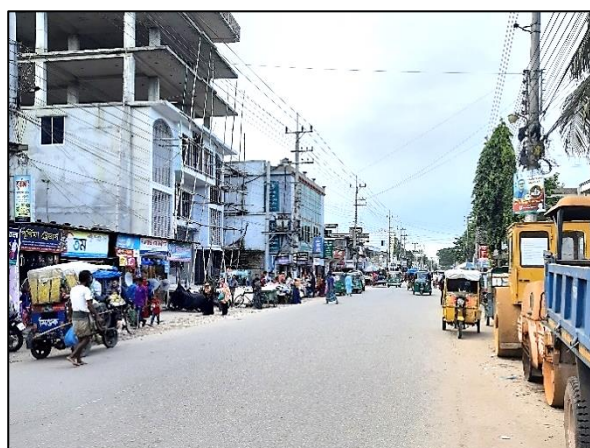
KULA-D-001: Improvement of road by Dense Bituminous Carpeting from Shibpur mour to Shibpur bridge & installation of Street Light 30 nos. at Ward no - 08, Kulaura Paurashava, Moulvibazar. Total Length = 860m
