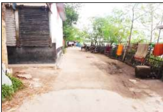
KUMA-R-003: Improvement of Road by DBC Starting From Public Library upto M.N. School Road. (Ch. 0+000 to 1+310) & installation of Street Light 44 nos. at ward no. - 03, Kumarkhali Paurashava, Kushtia. Total length = 1310m..
