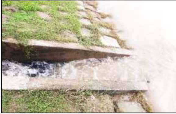
KUMA-D-019-Offfall: Construction of RCC Drain from Allonggi Para Adv. Kazol house to River Gorai via Matha Bhanga Mandir at ward no. - 03, Kumarkhali Paurashava, Kushtia. Total Length = 1119m
