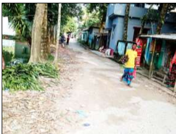
MADA-R-024: Improvement of Road by BC to RCC from Proshika office Mour Towards Madan - Kendra BC Road (Ch. 0.00m to Ch. 280m) & installation of Street Light 10 nos. at ward no. - 07, Madan Pourashava, Netrokona. Total Length = 280m..
