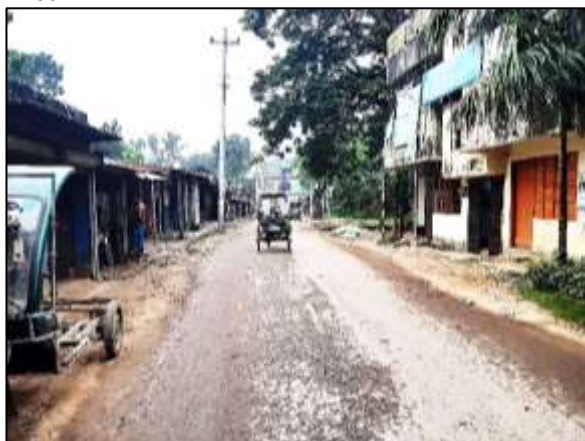
MADA-D-002: Construction of RCC Drain beside Madan - Natrona RHD Road (right and left side) from Dakbanglo near DC Road to Mogra River (Ch. 0.00m to 328m) (both sides) at Ward no. - 03, Madan Pourashava, Netrokona. Total Length = 656m..
