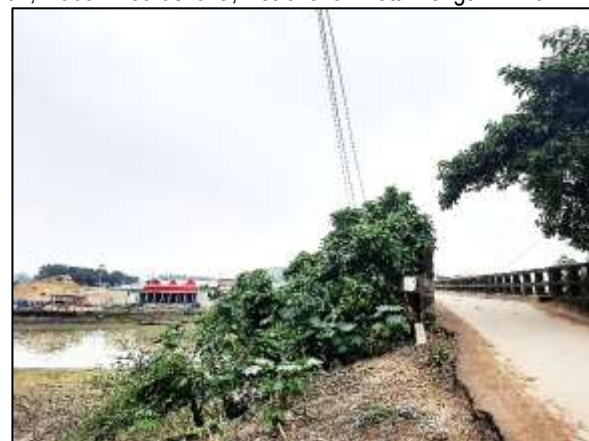
MADA-D-002-Outfall-Mogra River: Construction of RCC Drain beside Madan - Natrona RHD Road (right and left side) from Dakbanglo near DC Road to Mogra River (Ch. 0.00m to 328m) (both sides) at Ward no. - 03, Madan Pourashava, Netrokona. Total Length = 656m..
