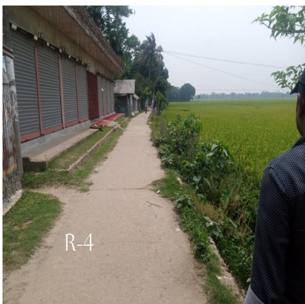
MADA-R-04: Construction of RCC Road Starting from Vari Vadera bridge mour towards water pump & Jewels House (Ch. 00to 654m) Total Length = 654m with 2 Nos. (X-drain-1.0x1.0m), Ch 00 to 56m & 287m & installation of Street Light 22 nos in Ward no. 04 Under Madan Pourashava, Netrokona.
