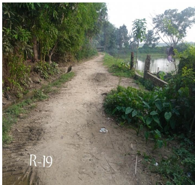
MADA-R-19 Construction of RCC Road Starting from Barobaroi road towards Ahmeds House via Roman's house (Ch. 00 to 229m) with 1 Nos. (X-drain-1.0x1.0m),Ch. 00 to 05m. Total Length = 229m with RCC palisading L=89m, & installation of Street Light 08 nos in Ward no. 05 Under Madan Pourashava, Netrokona.
