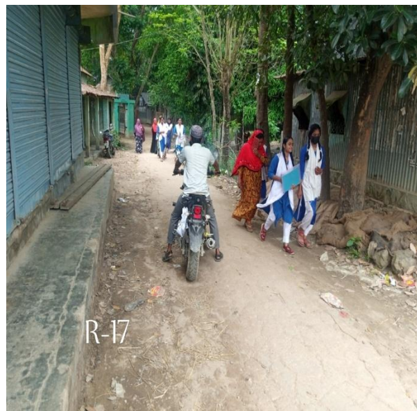
MADA-R-17: Construction of RCC Road Starting from Madan-Khaliyajury DC road towards Madan Thana road via Masterpara (Ch. 00 to 175m) & Link-1: Starting from Omol house to Madan Public High School (Ch. 00 to 60m),with 1 Nos. (X-drain-1.0x1.0m),Ch. 00 to 107m & installation of Street Light 9 nos Total Length = 235 in Ward no. 04 Under Madan Pourashava, Netrokona.
