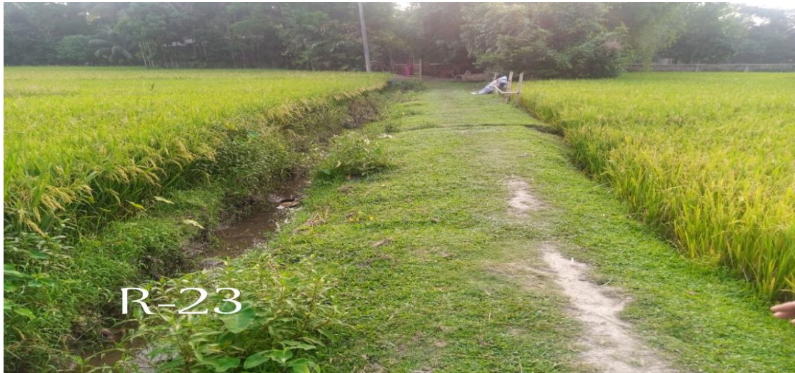
MADA-D-23: Construction of RCC Starting from with Road Development Madan – Fatepur Road to Mogra River via Popi Councilor's House (Ch.0.00-326.00m), at Ward No. 05 Under Madan Pourashava, Netrokona.
