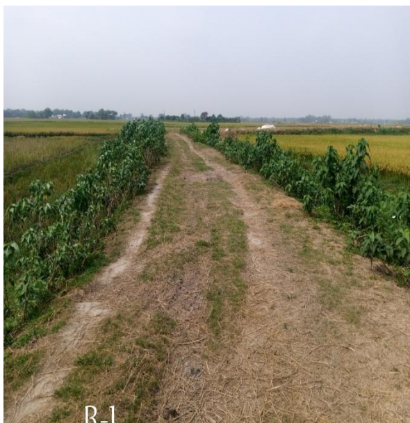
MADA-R-01: Construction of RCC Road Starting from Hafija Madrasa towards Kha-Bil (Ch.00 to 1000m) Total Length = 1000m with 4 Nos (1V-4.5x4.5), Ch at 00 to 70m, 335m, 496m & 627m. Box culvert & installation of Street Light 34 nos in Word no. 01 under madan pourashava, Netrokona.
