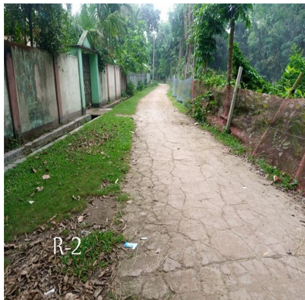
MADA-R-02: Construction of RCC Road Starting from Moulo Mias Shop towards Haruns house Via Shafique Councilors house Part-A (Ch. 00 to 490.00m) & installation of Street Light 17 nos With 3 Nos (X-Drain -1.0X1.0m), Ch. 102m, 176m & 295m Total Length =490.00m in Word no. 01 under madan pourashava, Netrokona.
