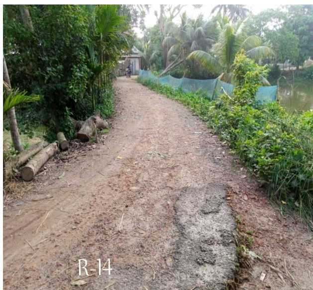
MADA-R-14: Construction of RCC Road Starting from Liton Chairmans House mour towards Mazar Mosque Road via Jholmol's House (Ch. 00 to 415m) with four link road, link -1: Starting from Aulat hussain house to Madan-Khaliyajury road (Ch. 00 to 192m), Link- 2: Starting from Indrojit house Madan Khaliyajury road (Ch. 00 to 187m), Link-3 : Starting from Narayon Councilor to Madan Khaliyajury road (Ch. 00 to 173m), Link- 4: Starting from Ram Krishno mondir opposite to Madan Fotehpur road (Ch. 00 to 300m), 65m Protection Work & installation of Street Light 44 nos, Total Length = 1267 with 5 Nos. (x-drain -1.0x1.0m),Ch. 00 to 105m,195m,235m,248m & 362m. In Ward no. 04 Under Madan Pourashava, Netrokona.
