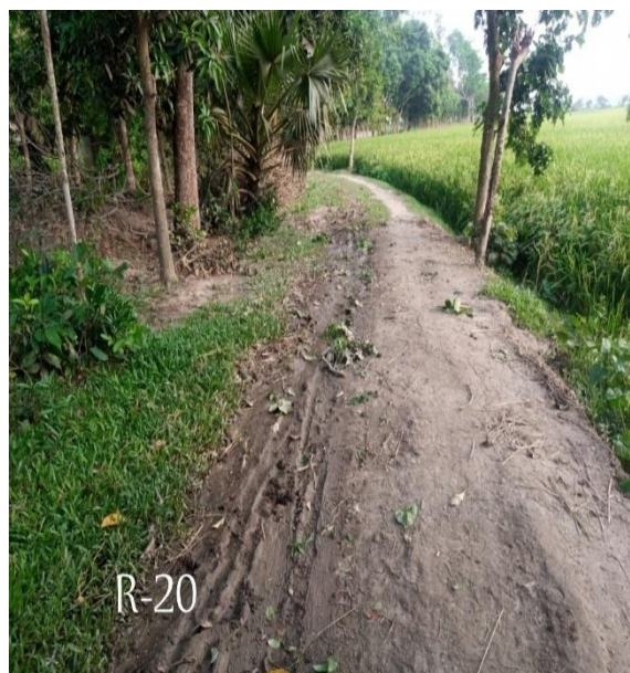
MADA-R-20 Construction of RCC Road Starting from Barobaroi road towards Jahid's house (Ch. 00 to 289m), with 1 Nos. (X-drain-1.0x1.0m),Ch 00 to 05m & installation of Street Light 10 nos Total Length = 289m in Ward no. 05 Under Madan Pourashava, Netrokona.
