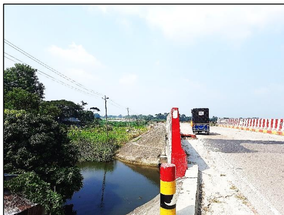
MATL-D-021-Outfall: Improvement of road by RCC from Baghar Khal to Choughoria road including RCC Box Culvert at Ch. 850m, Protection Work & installation of Street Light 30 nos. at Ward no - 9, Matlab Pourashava, Chandpur. Total Length = 875m.
