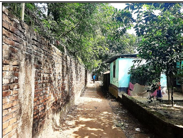
MATL-R-024: Improvement of road by Dense Bituminous Carpeting from Jhoughora to Mozzakanda Bazar including of Protection Work at (Ch. 0m to 55m, L/S), (Ch. 225m to 250m, L/S), (Ch. 320m to 360m, L/S), (Ch. 650m to 700m, L/S) & installation of Street Light 40 nos. at Ward no - 2 & 5, Matlab Pourashava, Chandpur. Total Length = 1181m.
