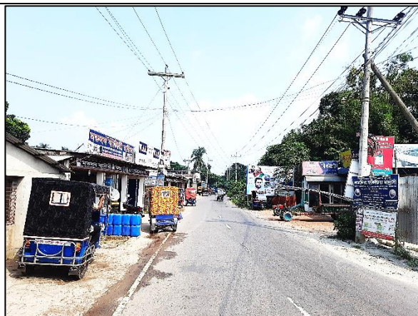
MATL-D-021: Improvement of road by RCC from Gazipura Fish Hatchery Main Road to Gazipura North Para Eidgah Road including Protection Work at (Ch. 230m to 250m, L/S) & installation of Street Light 9 nos. at Ward no - 6, Matlab Pourashava, Chandpur. Total Length = 250m.
