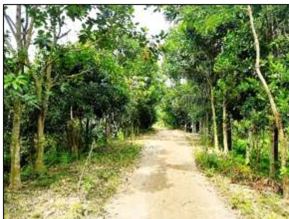
R-012: Improvement of road by Dense Bituminous Carpeting from North Baispur Graveyard to Hamid Mirdha house via Secretary Abul Hossain house (Ch. 0.00m to 1327m) at Matlab Pourashava, Ward no - 01, Chandpur. Total Length = 1327m
