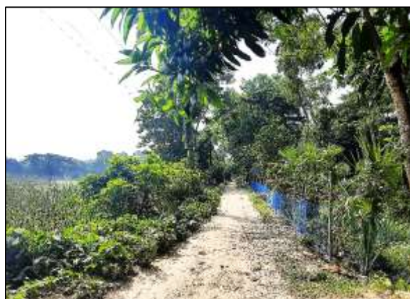
R-021: Improvement of road by Dense Bituminous Carpeting from Roic Miazi house to Middle Digoldi Nanto Gazi house (Ch. 500.00m to 1500m) including Protection Work at (Ch. 1400m to Ch. 1450m, L/S) at Matlab Pourashava, Ward no - 06, Chandpur. Total Length = 1000m..
