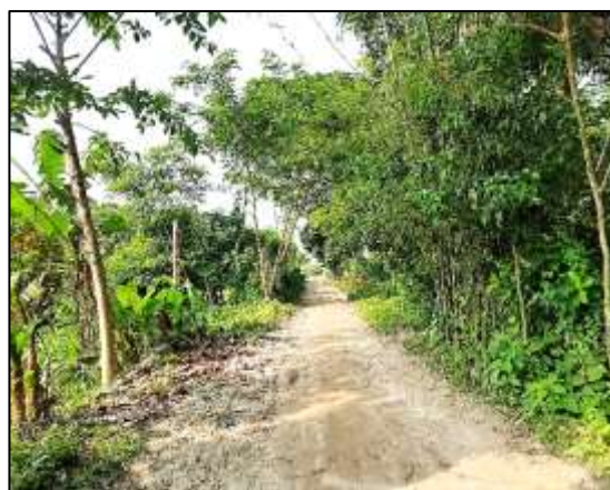
Improvement of road by Dense Bituminous Carpeting from Bari Nagar to towards Algrimukundi Bridge (Ch. 0.00m to 1300.00m) including Protection work at (Ch. 80m to 230m, R/S, Ch 1050-1100m Both side & Ch 1225m to 1300m) at ward no - 05, Matlab Pourashava, Chandpur. Total Length = 1300m.
