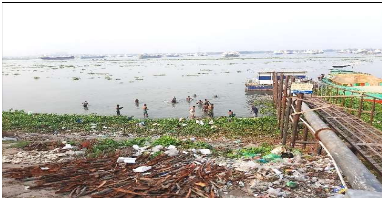
MUNS-D-027-Outfall: Construction of RCC Drain from Hatlakhmiganj Madrasa to Dhaleshwari River via WTP (Ch. 0.00m - Ch. 235.00m), at Ward no.- 3, Munshiganj Paurashava, Munshiganj. Total Length = 235.00m
