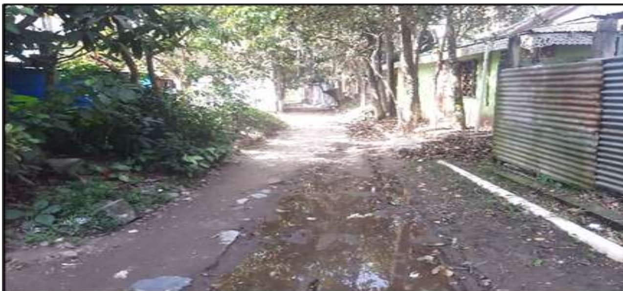
MUNS-R-036: Improvement of Road by Reinforced Cement Concrete (RCC), starting from Dewbhog Graveyard to h/o Mozibur Chairman at Dewbhog (Ch. 0.00m - Ch. 704.00m), at Ward no.- 4, Munshiganj,. Total Length = 704m.
