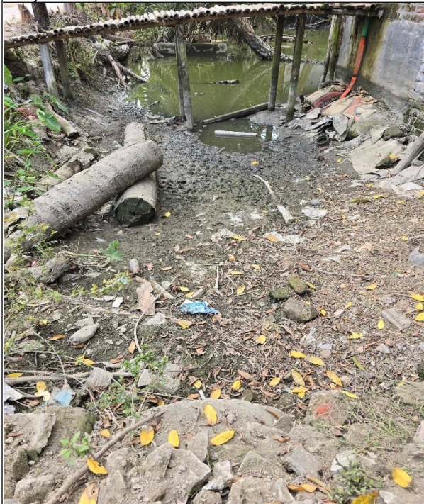
D-276- Construction of RCC Drain starting from Vogruil Graveyard to existing drain (Ch.250 to 475m), Total Length=225m under Naohata Paurashava, District Rajshahi
