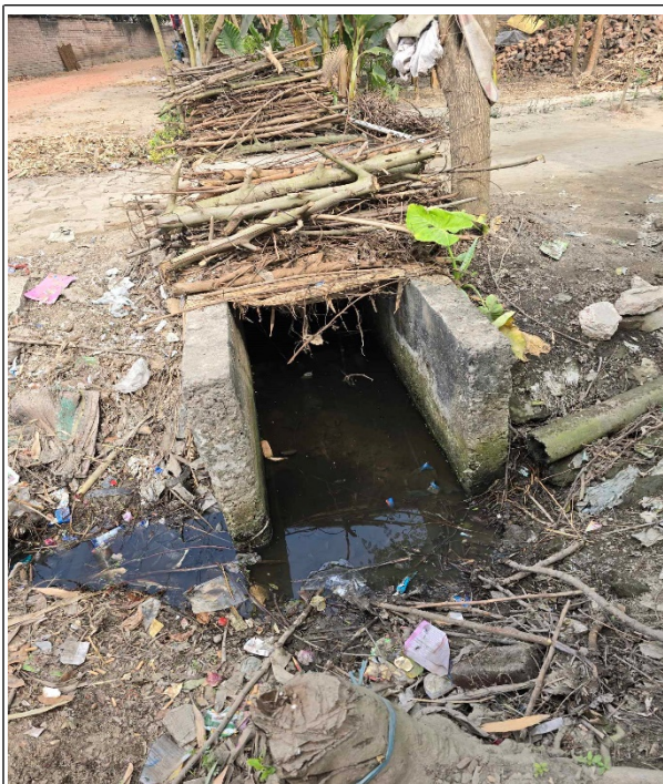
D-272- Construction of RCC Drain starting from Vogruil Dalan to existing Bathan Bari Outfall Part-A,(Ch.538 to 1169m) & Part-B,(Ch.100 to 375m) Total Length=906m under Naohata Paurashava, District Rajshahi.
