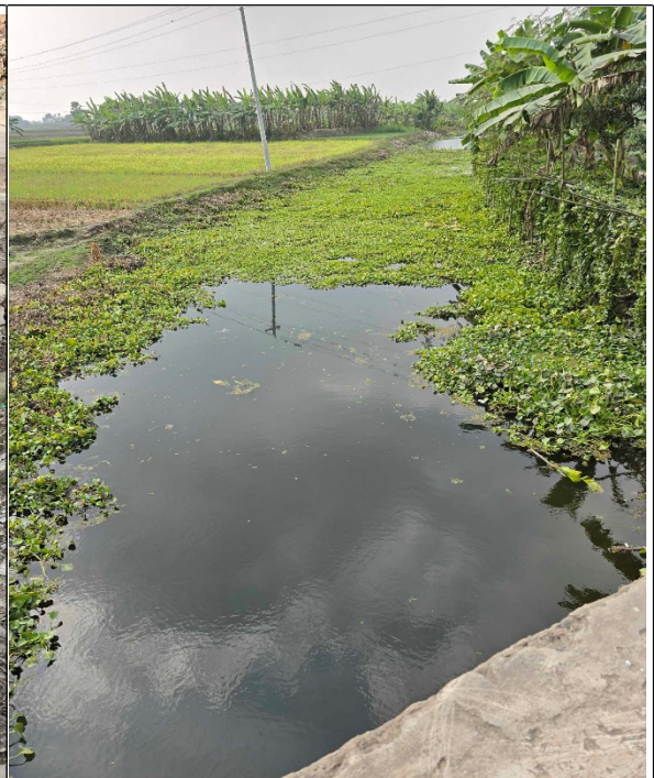
D-342- Construction of RCC Drain from near Shialbed house of Zoban existing RCC Drain to Doyar Bridge (Doyar Shaku Canal) (Ch.550 to 895m), Total length = 345m under Naohata Paurashava, District Rajshahi.
