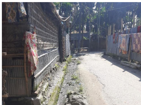
PATG-D-001: Construction of RCC Drain, starting from Aminur's Farm to Proposed Drain D-002 near Jhakuatari Mosque (Ch. 0.00m - Ch. 100.00m) and from Sofikar's house to Proposed Drain D-002 near Jakuatari Mosque (Ch. 0.00m - Ch. 200.00m), at Ward no.- 2, Patgram Paurashava, Lalmonirhat. Total Length = 300m.
