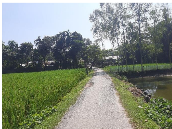
PATG-R-007: Improvement of Road by Dense Bituminous Carpeting (DBC), starting from Munsirhat BC Road to the North side of Aminur Mia's Farm (Ch. 0.00m - Ch. 616.00m), including RCC Cross Drain at Ch. 500m and Protection Works at (Ch. 150m to Ch. 220m, L/S), at Ward no.- 2, Patgram Paurashava, Lalmonirhat. Total Length = 616m.
