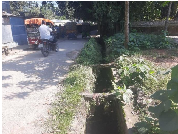
PATG-D-008: Construction of RCC Drain starting from Posu Hospital to the existing drain near Abu Bakkar Siddik's house (Ch. 0.00m - Ch. 396.00m), at Ward no.- 5, Patgram Paurashava, Lalmonirhat. Total Length = 396m.
