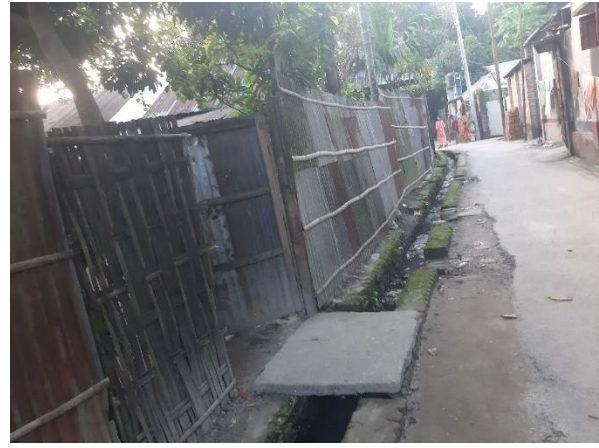
PATG-D-010: Construction of RCC Drain starting from Rolex House to the existing drain near Labu Sangbadik's house via Poura BC Road Mour (Ch. 0.00m - Ch. 210.00m) and Link Drain from Rail Line to Paura BC Road Mour (Ch. 0.00m - Ch. 47.00m), at Ward no.- 5, Patgram Paurashava, Lalmonirhat. Total Length = 257m.
