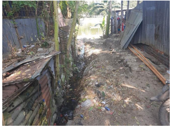
PATG-D-011: "Construction of RCC Drain, starting from Hamidul's House to Dharla River via Aminur's shop (Ch. 0.00m - Ch. 232.00m) and Link Drain from Rokan's house to Aminur's shop (Ch. 0.00m - Ch. 75.00m), at Ward no.- 6, Patgram Paurashava, Lalmonirhat. Total Length = 307m."
