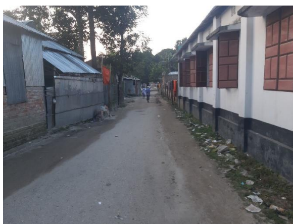
PATG-D-018: Construction of RCC Drain, starting from Station Road to the existing drain near Patgram Bypass RHD Road (Ch. 0.00m - Ch. 363.00m) and Connecting Drains (a) from Jobaidul's house to Hob's house via Shahin's house (Ch. 0.00m - Ch. 250.00m) & (b) from Fozol Bihari's house to Habib's Shop (Ch. 0.00m - Ch. 160.00m), at Ward no.- 8, Patgram Paurashava, Lalmonirhat. Total Length = 773m.
