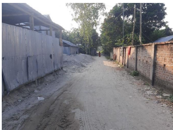
PATG-R-035: Improvement of Road by Dense Bituminous Carpeting (DBC), starting from Lalmonirhat RHD Road to Soreo Bazar (Ch. 0.00m - Ch. 1250.00m), including Protection Works at (Ch. 80m to Ch. 320m, L/S), (Ch. 470m to Ch. 540m, R/S) & (Ch. 720m to Ch. 770m, L/S) and installation of Street Lights of 43 nos., at Ward no.- 9, Patgram Paurashava, Lalmonirhat, Total Length = 1250m.
