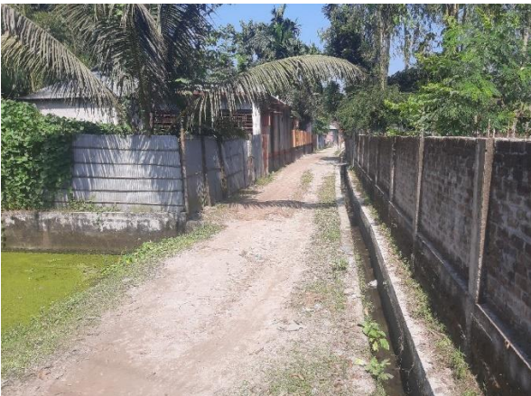
PATG-R-027: "Improvement of Road by Reinforced Cement Concrete (RCC), starting from Rail Station Road to Patgram Bypass RHD Road (Ch 0.00m - Ch. 476.00m), including installation of Street Lights of 17 nos., at Ward no.- 8, Patgram Paurashava, Lalmonirhat. Total Length = 476m."
