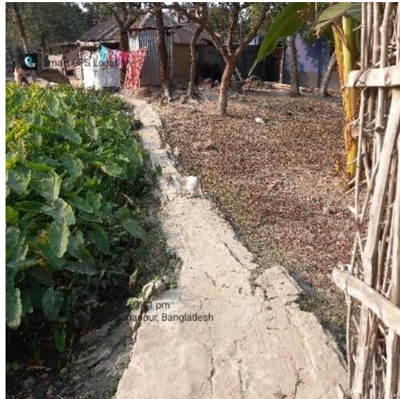
Figure IV.9: Existing Situation of Footpath at Gombujpara LIN
