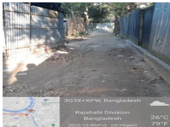
Figure IV.3: Existing Situation at Bohipara Daingpara LIN
