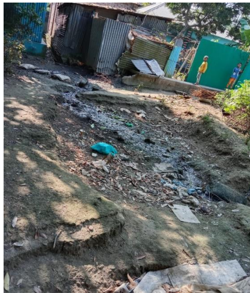
Figure IV.4: Existing Situation of Drain at Bohipara Daingpara LIN
