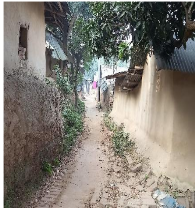
Figure IV.1: Existing Situation of Footpath at Rohanpur School para-LIN
