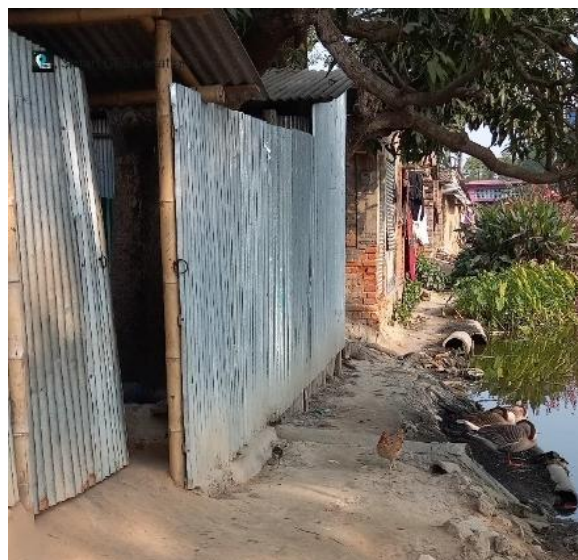
Figure IV.10: Existing Situation of Drain at Gombujpara LIN
