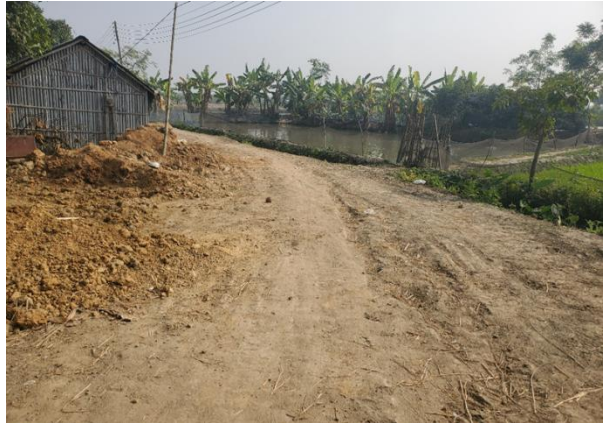
Existing Earthen Road at ch 200m
