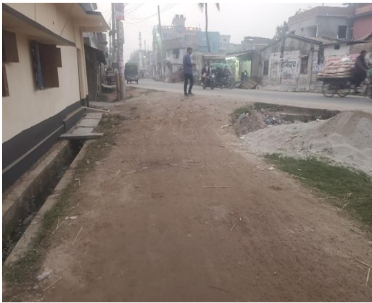
Existing BC Road at ch 10m
