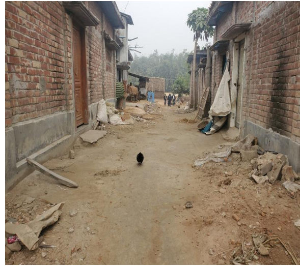
Existing Earthen Road Link, at ch 40m
