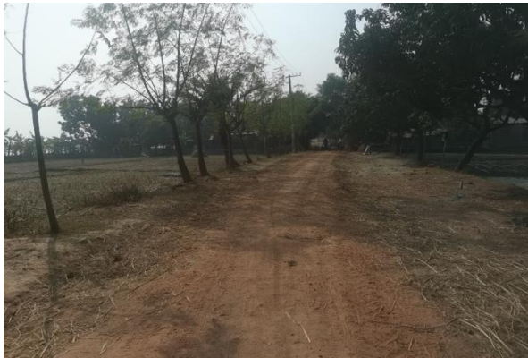
Existing Earthen Road at ch 35m
