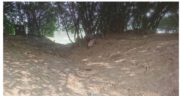
Existing Earthen Drain at ch.1030m (Outfall)
