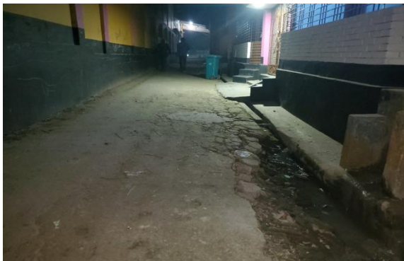
Existing Earthen drain at ch 95m
