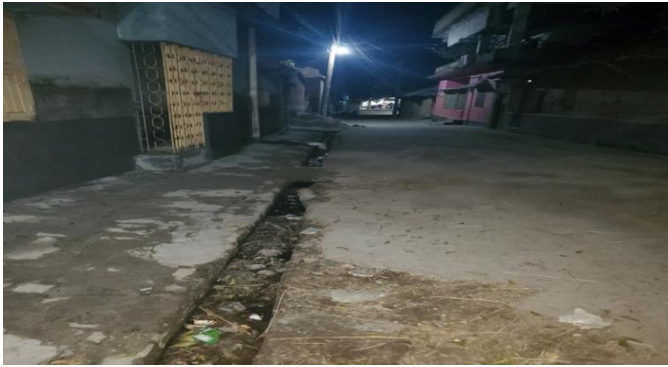
Existing CC Road at ch 110m
