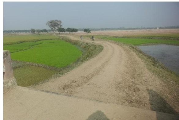
Existing Earthen Road at ch 900m
