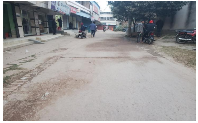
Existing Earthen Drain Link, at Ch.
