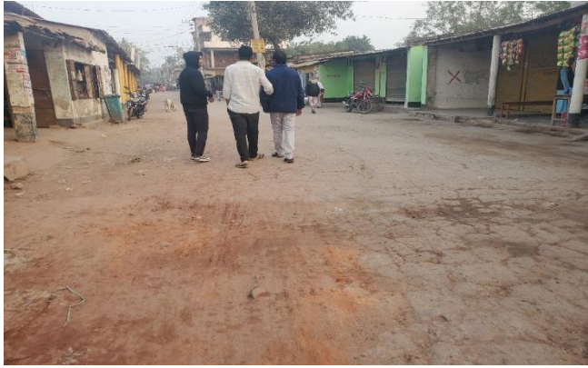
Existing Earthen Drain at ch.95m 120m
