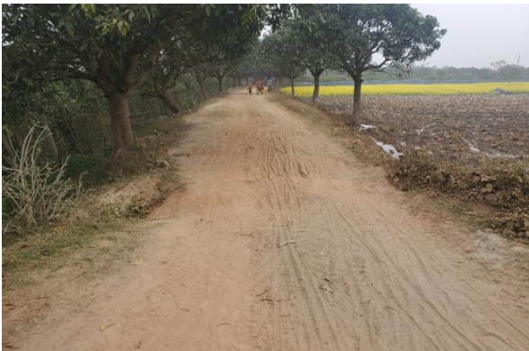
Existing Earthen Road Link, at ch 25m
