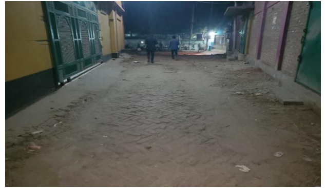
Existing CC Road at ch 155m
