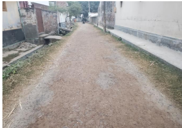
Existing BC Road at ch 120m
