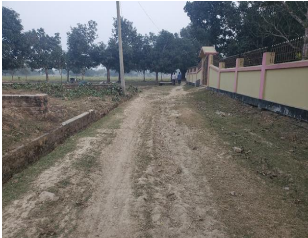
Existing Earthen Road at ch 350m
