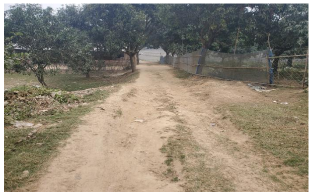
Existing Earthen Road at ch 40m
