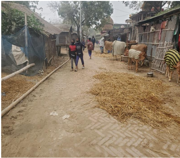
Existing HBB Road at ch 45m
