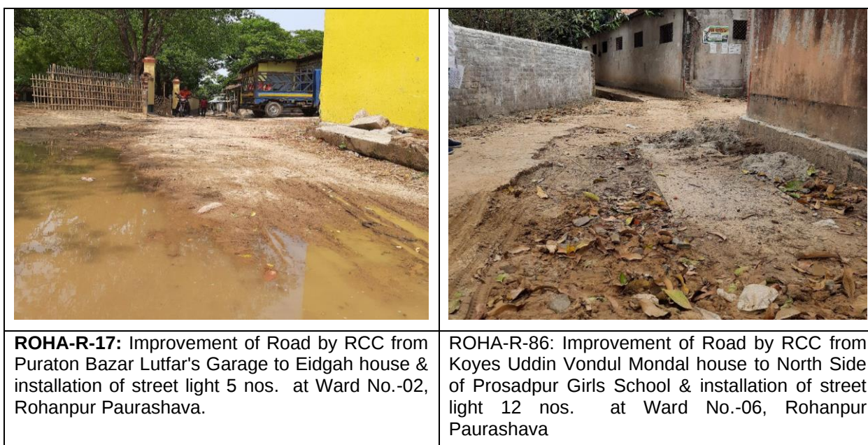
Figure IV.3: Existing Conditions of Paurashava Road
