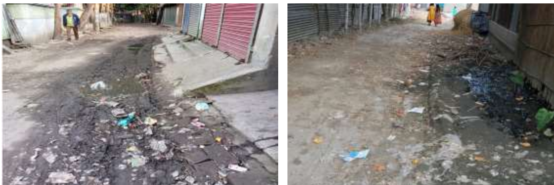
Figure 3: Existing condition of roads & drains
