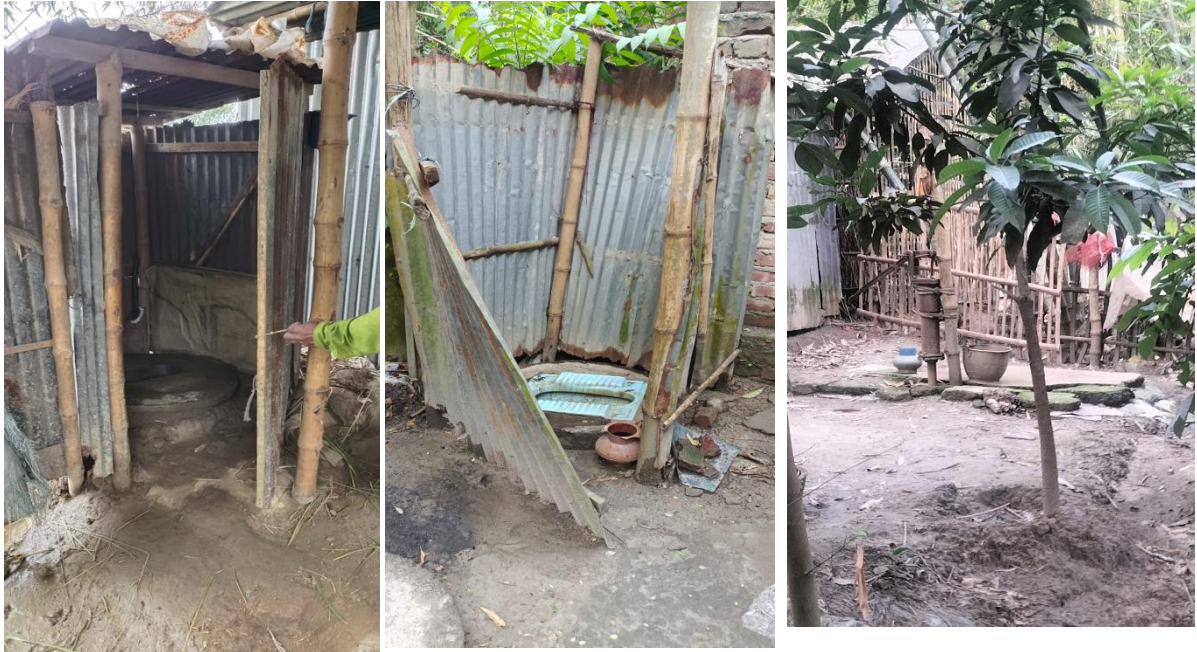
Figure IV.4: Existing Situation at Dokkhin Baroipara LIN
