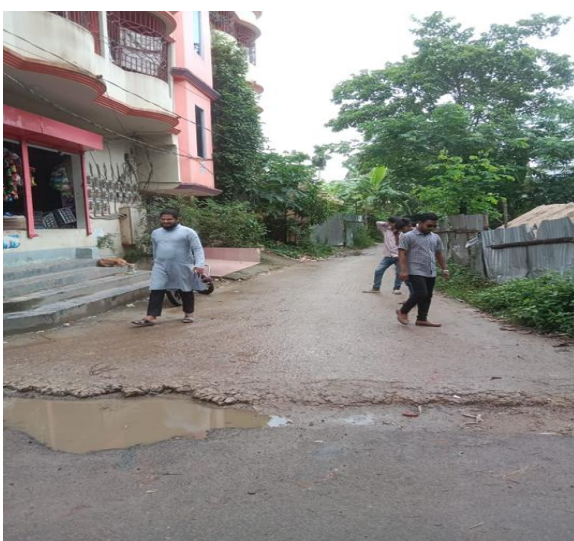
SP.RD8.002: Improvement of Road starting from Kasem Store and ending near Selim Tower (Ch.0+00km to 0+592.00km) & by RCC Road, including Protection work 60m at with 21 nos Street Light at ward no-08 under Sonagazi Pourashava, District Feni; Total Length = 592.00m.
