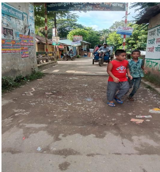
SP.RD3.001: Improvement of Road by Uni-Block Paver & RCC starting from Engr. Masud Bari and ending near South Patowary Bari, Uni-Block Paver (Ch.0.00-325.00m & Ch. 770.00-1160.00m), RCC (Ch. 325.00-770.00m), Installation of 39 Nos. Street Light at ward no-03 under Sonagazi Pourashava, Feni. (Total Length=1160.00m).
