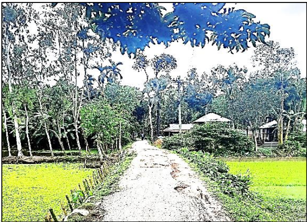
ULIP-R-10: Improvement of road by Dense Bituminous Carpeting from Purbo Shibbari Bazar to Aziz Bepari house of Pakhimaritari (Ch. 0.00m to 1248m) including Protection Work & installation of Street Lights 43 nos. at Ward no. - 05, Ulipur Paurashava, Kurigram. Total Length = 1248m.
