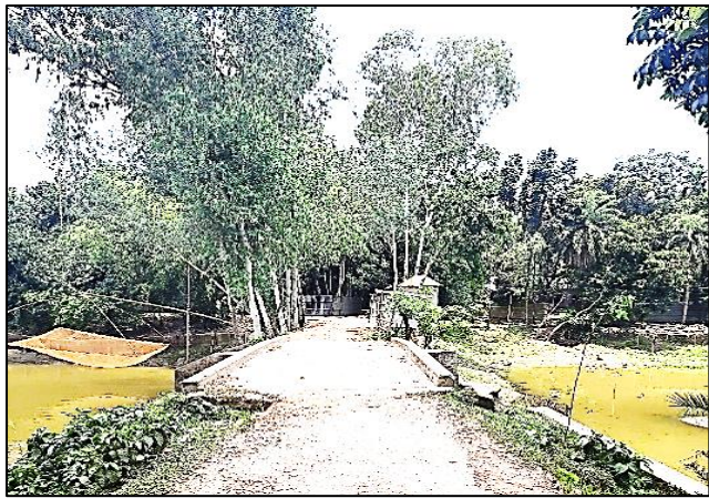
ULIP-R-01: Improvement of road by RCC & DBC from Dr. Nazma house front road to Khamar Govt. Primary School Road (Ch. 0.00m to 2020.00m) including Protection Work & installation of Street Lights 68 nos. at Ward no. - 03, 04 & 06, Ulipur Paurashava, Kurigram. Total Length = 2020m.
