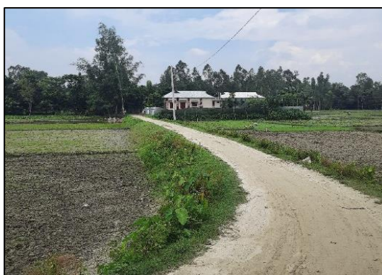
ULIP-R-15: Improvement of road by Dense Bituminous Carpeting from Paglakura Eid-Gah-Math to Hayat Khan Govt. Primary School Road including RCC Cross Drain, Protection Work & installation of Street Light 24 nos. at Ward no.-3, Ulipur Pourashava, Total Length = 675m.
