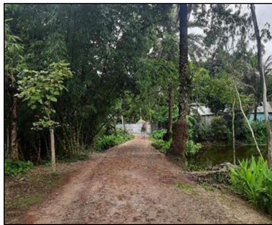
ULIP-R-09: Improvement of road by Dense Bituminous Carpeting from Malotibari Bazar Road to Milon house via Engineer Malek house road including RCC Box Culvert, RCC Cross Drain at Ch. 1144m, Protection Work & installation of Street Light 55 nos. at Ward-5, Ulipur Pourashava, Kurigram. Total Length = 1608m.
