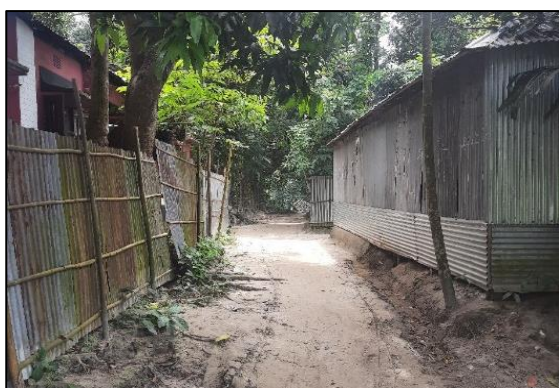
ULIP-R-012: Improvement of road by Dense Bituminous Carpeting from Miah Para Mour to Fasidah Bridge Road (Ch. 0.00m to 970m) including RCC Cross Drain at Ch. 291m, Ch. 613m, Protection Work & installation of Street Light 33 nos. at Ward no. - 1, Ulipur Pourashava. Total Length = 970m.
