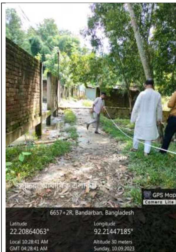
MP ID-AR566: Construction of RCC Road cum Drain Starting from Balaghata Basundhara Resedential area Sona Miya House to Mozafar House ward No-02 Under Bandarban Pourashava ( Ch:0.0-220m).
