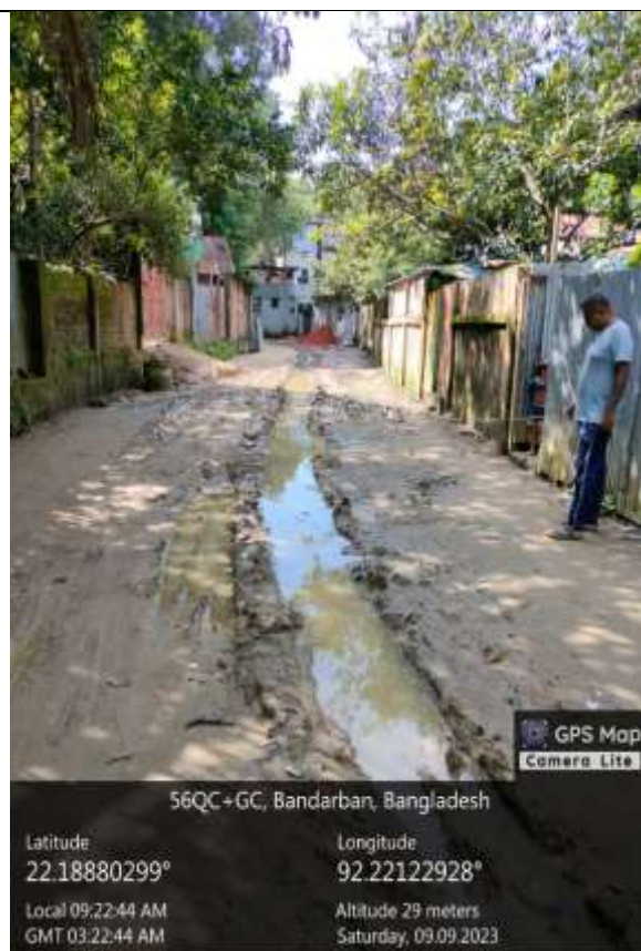
MP ID- AR624: Construction of RCC Road Starting from Stadium Road Islami Siksha Kendra to Muslim house road at Banarupa (Sibu Das House) ward no 06 under Bandarban Pourashava( (Ch:00-420m).
