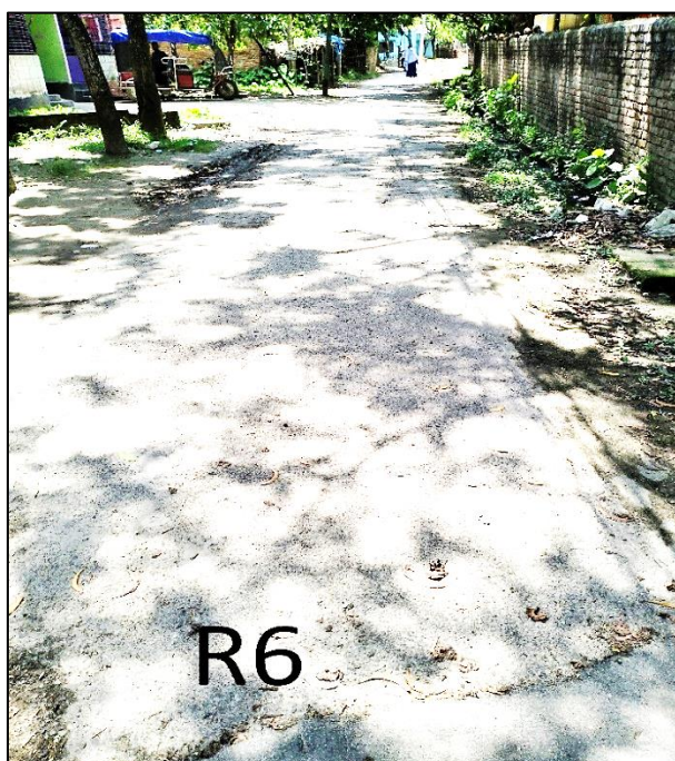
BHER/R-06: Improvement of road by Dense Bituminous Carpeting from Hazi Johir Uddin road (Ch. 0.00m to 590m) & installation of Street Light 21 nos. at Ward no. - 4, Bheramara Paurashava, Kushtia. Total Length = 590m.
