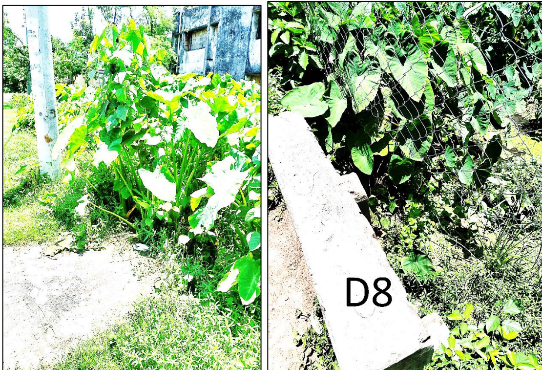
BHER-D-08: . Construction of RCC Drain from Sub zonal Office to Syphone of BWDB at Farakpur Ward No. - 02 & 03, (Ch.0.00m to 718m), Bheramara Paurashava, Kushtia. Total Length = 718m
