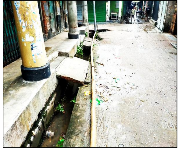
Drain- 23, Kumarkhali Pourashava
