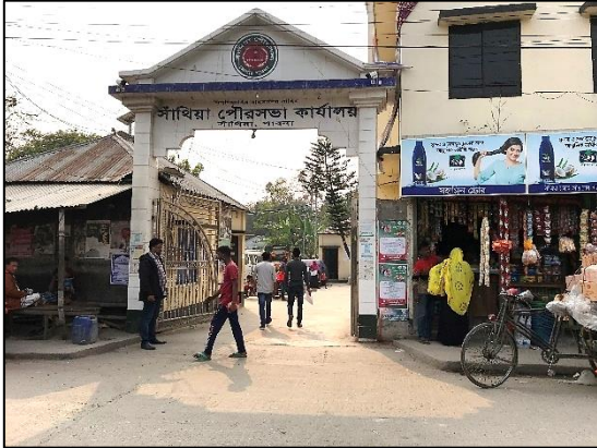
WARD-5: Main Gate surrounded by Santhia Bazaar shops.:..Proposed Santhia Paurashava Super Market on Paurashava partly old building and CI sheet roofing premise-at Santhia Bazar,
